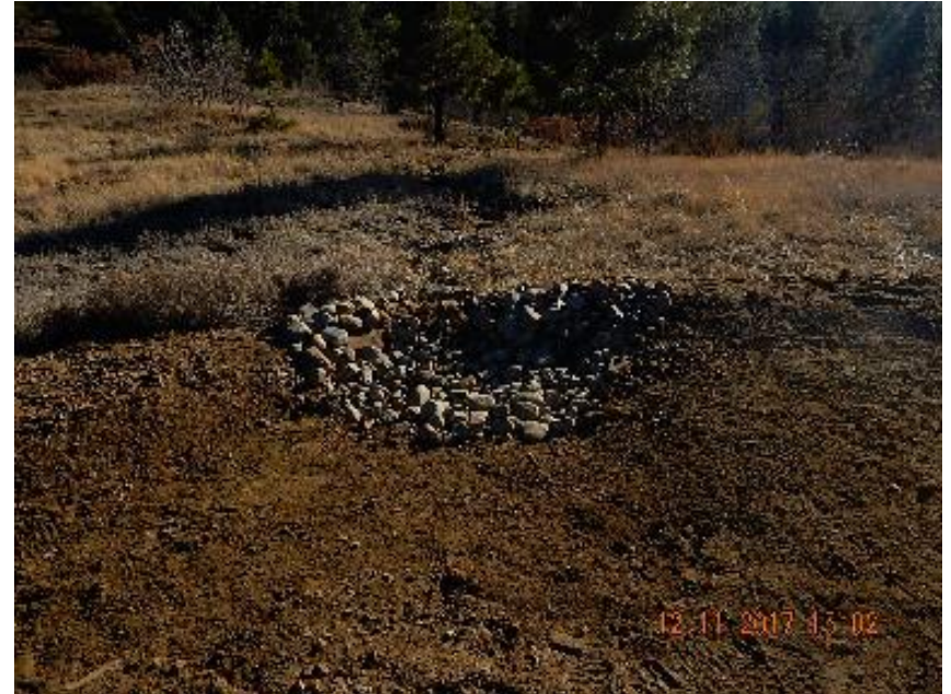
Photo 4: Sediment trap and rock run down on edge of location.
