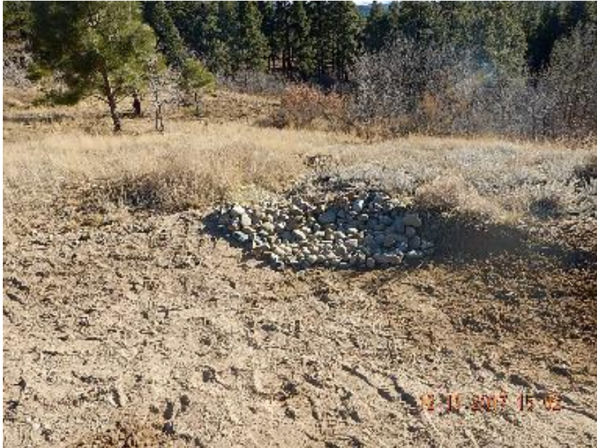
Photo 3: Sediment trap and rock run down off edge of location.
