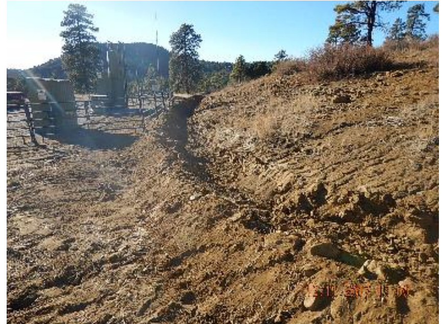
Photo 2: Ditch and berm along bottom of fill slope.
