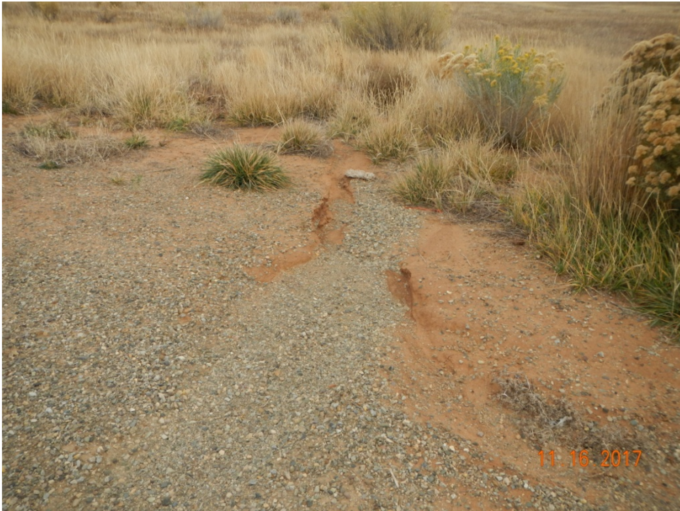
Photo 5. View of stormwater controls at the entrance to the well pad.
