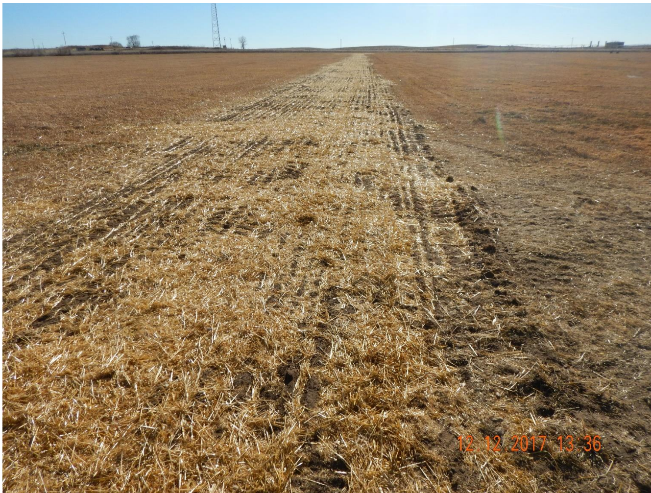
Photo 1: Photo taken from the access road, facing south. Photo shows road appears to have been seeded, and crimped with straw for stabilization.
