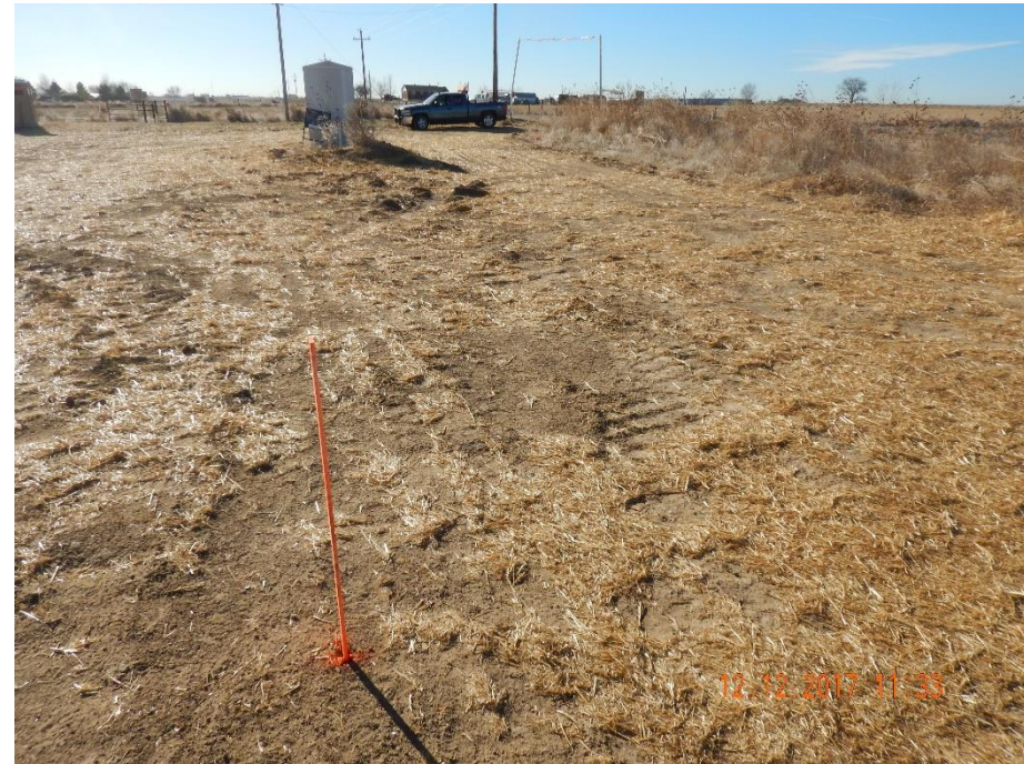
Photo 2: Photo taken from the north end of the tank battery location, facing southwest. Photo shows the majority of the location appears to have had additional reclamation work conducted, however, photo also shows meter shed equipment has not been removed per the corrective action.
