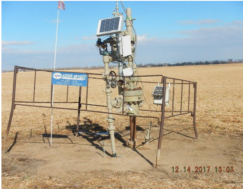
Photo 1 Wellhead API 05-123-16687 from south
