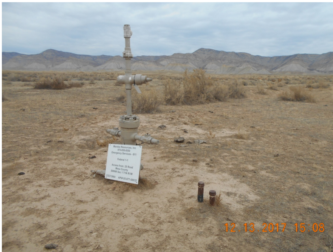
Wellhead with unused/unmarked risers
