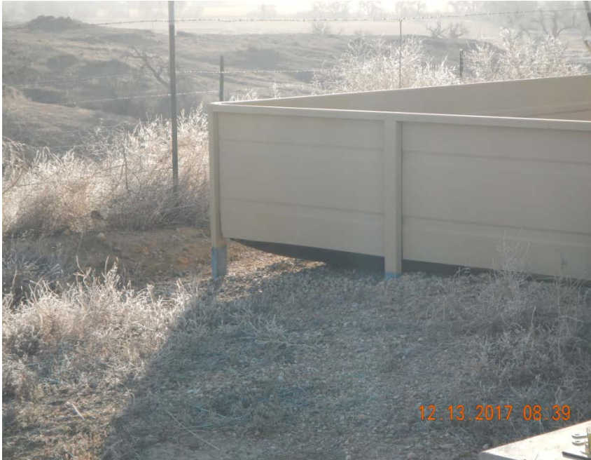
Crude oil tank berm and liner
