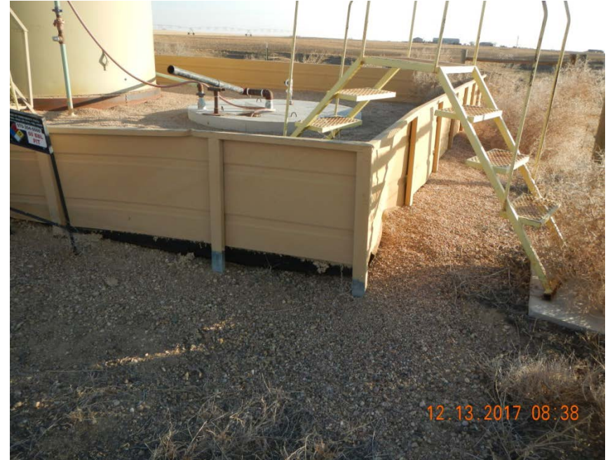
Crude oil tank berm and liner
