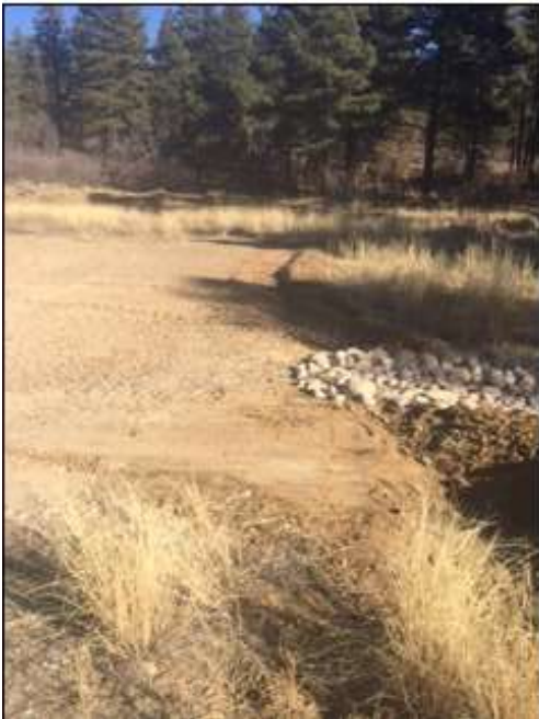
Rock run down installed to slow velocity and filter sediment of storm water flow off pad
