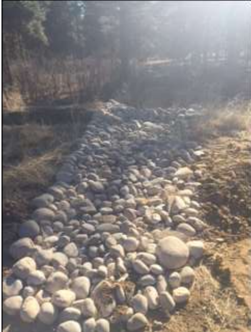
Rock run down installed armouring erosion channel to slow velocity and filter sediment of storm water flow off pad
