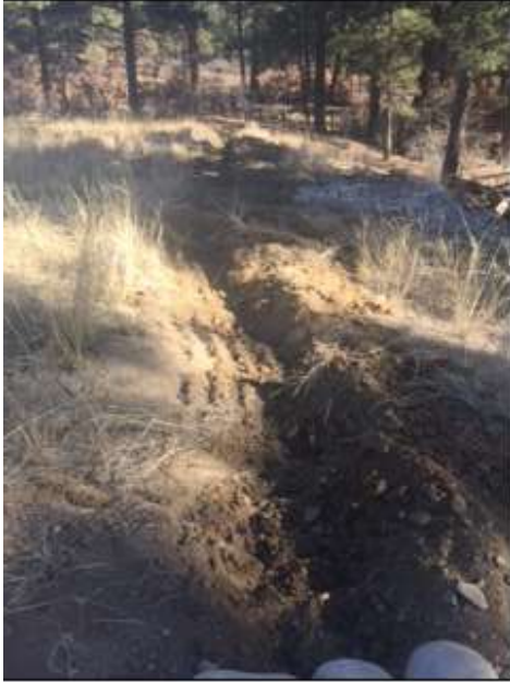
Diversion ditch on toe of slope installed to direct stormwater to the rock run downs to prevent future erosion channels
