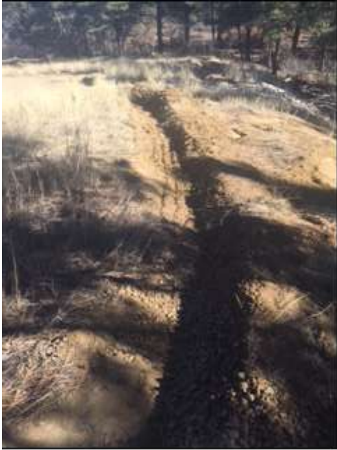
Diversion ditch around toe of slope to direct storm water flow to rock run down
