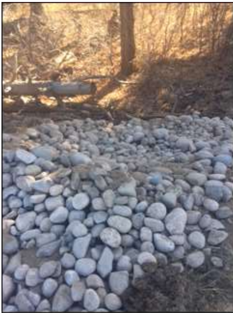
Second rock run down with check dams installed for armouring erosion channel to slow velocity and filter sediment of storm water flow off pad
