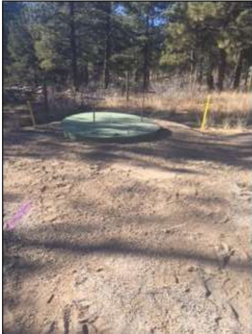
Additional photo of back fill around valve can
