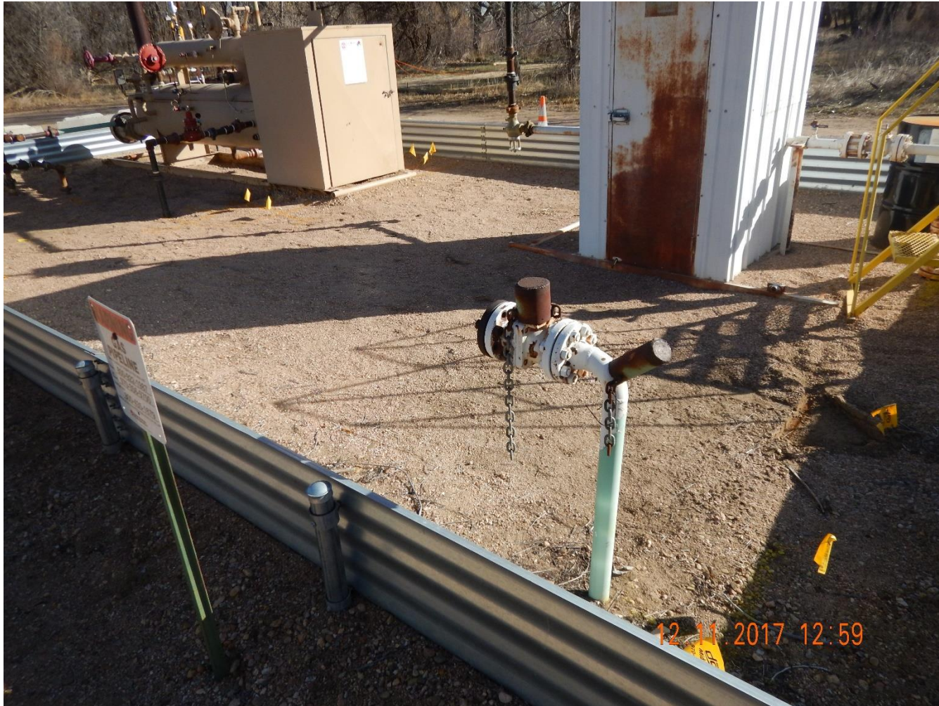
Photo 1: Photo taken from the battery facility. Previous inspections required operator to remove abandoned gathering riser in accordance to COGCC reclamation rule 1004.a. Photo shows riser has not been removed.
