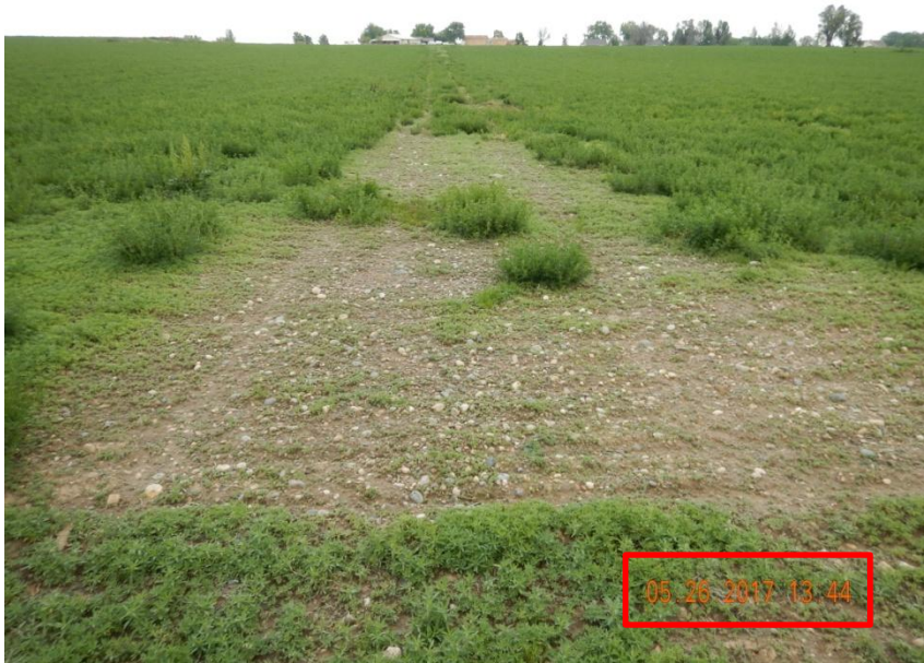
Photo 1. Photo taken on May 26, 2017 from the access point off CO Rd. 16, facing North along the access road. Gravel has not been removed and access road has not been contoured.
