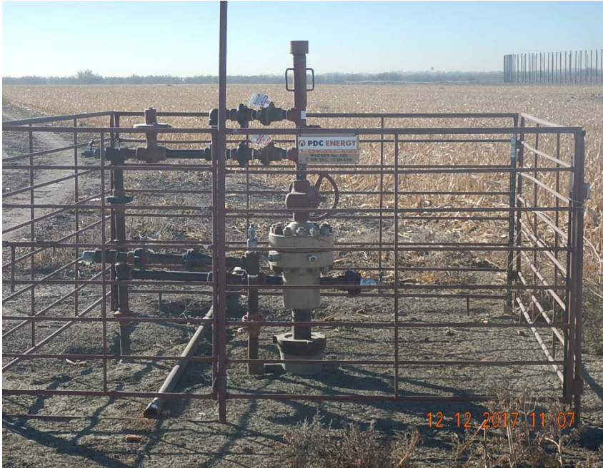
Photo 1: Wellhead, looking SW
