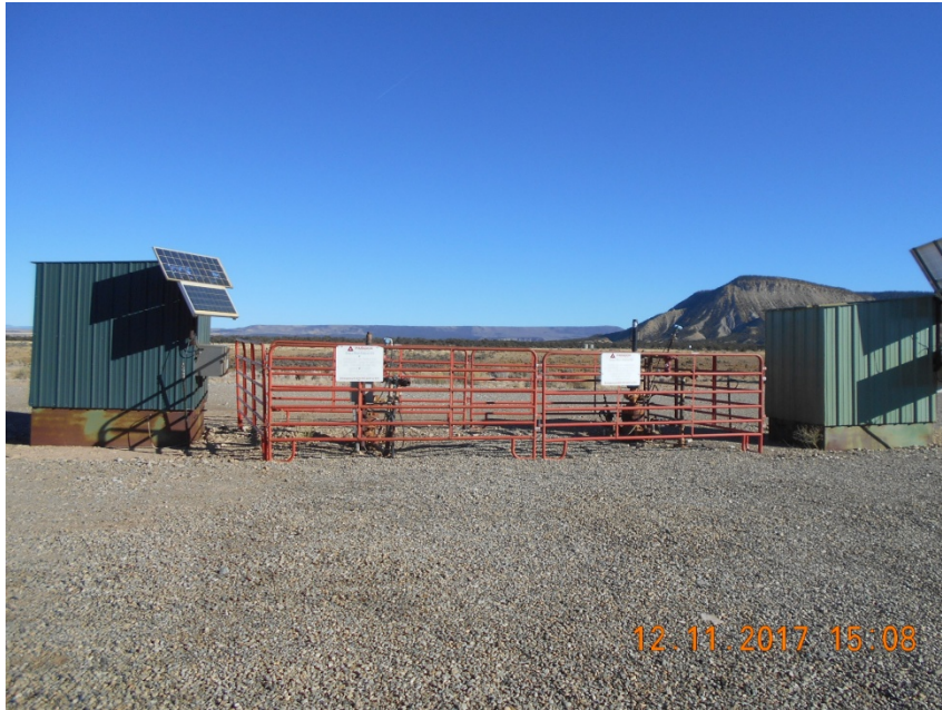
Wellheads with fencing and signs.
