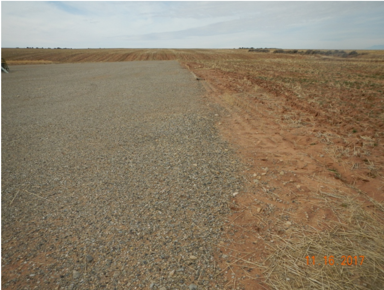
Photo 2. View of the northern portion of the project area from the northeastern corner facing westward. Well pad size is reduced and interim reclamation areas are incorporated into surrounded cropland. Vegetation in disturbance areas should be monitored in comparison to reference vegetation.
