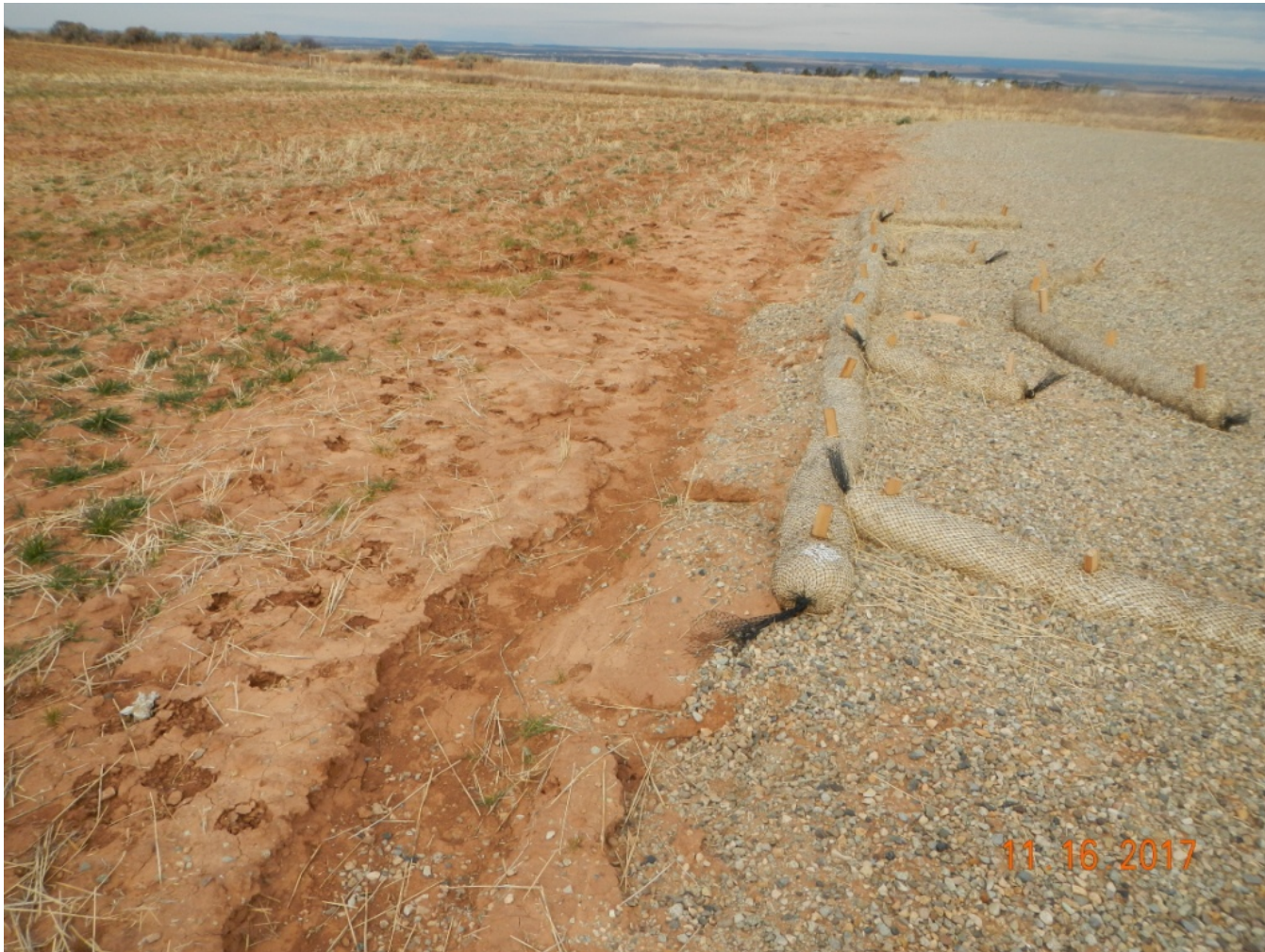
Photo 4. View of wattles in the western portion of the project area. These appear to need maintenance, and do not appear to be sufficient length to prevent concentrated runoff from the well pad eroding adjacent crop soils.
