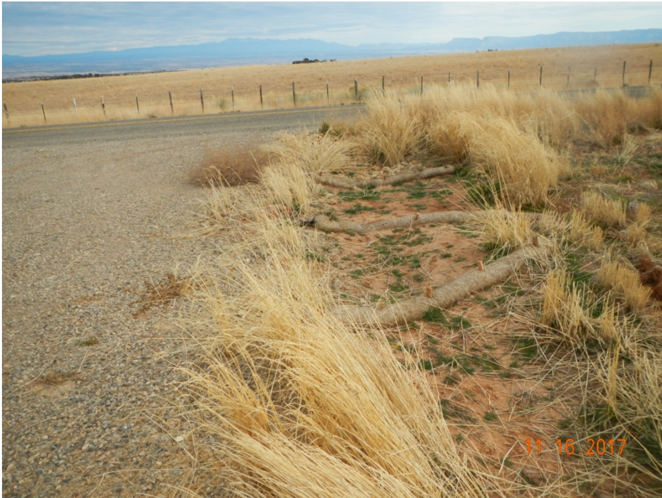
Photo 6. View of wattles along the southern portion of the access road, appear to be functioning.
