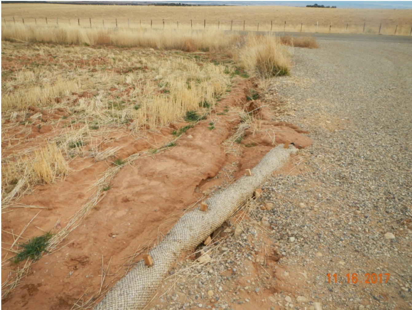
Photo 5. View of wattle at the entrance to the well pad, needs maintenance.
