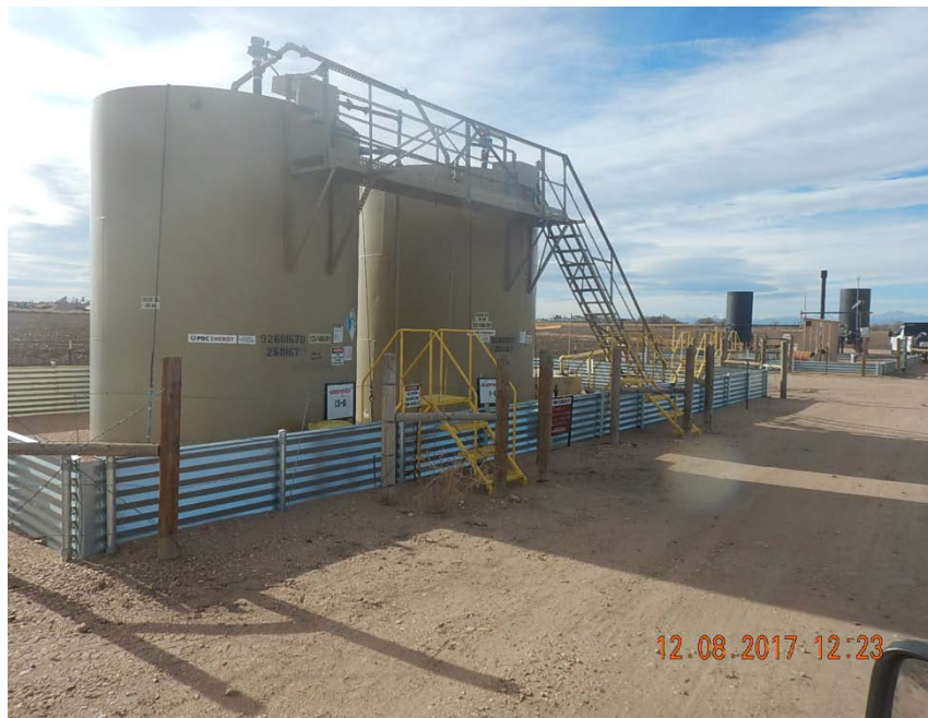
Photo 1: Location, looking SW
