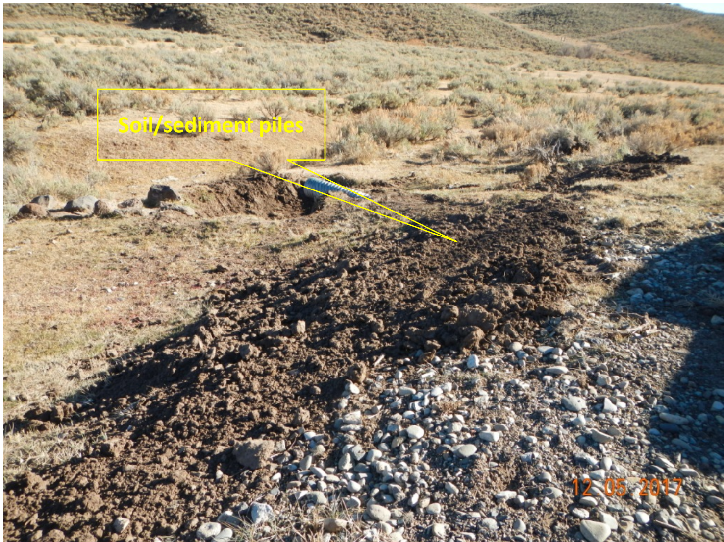
Photo 4. View of area along the access road where sediment and soil has been scraped and placed in piles along roadside and in adjacent grass/sagebrush habitats.
