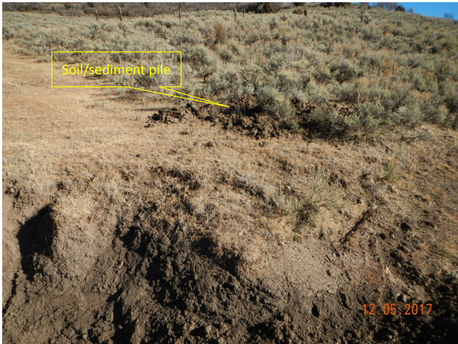
Photo 1. View of area along the access road where silt trap was recently cleaned and sediment placed offsite into adjacent sagebrush habitat.
