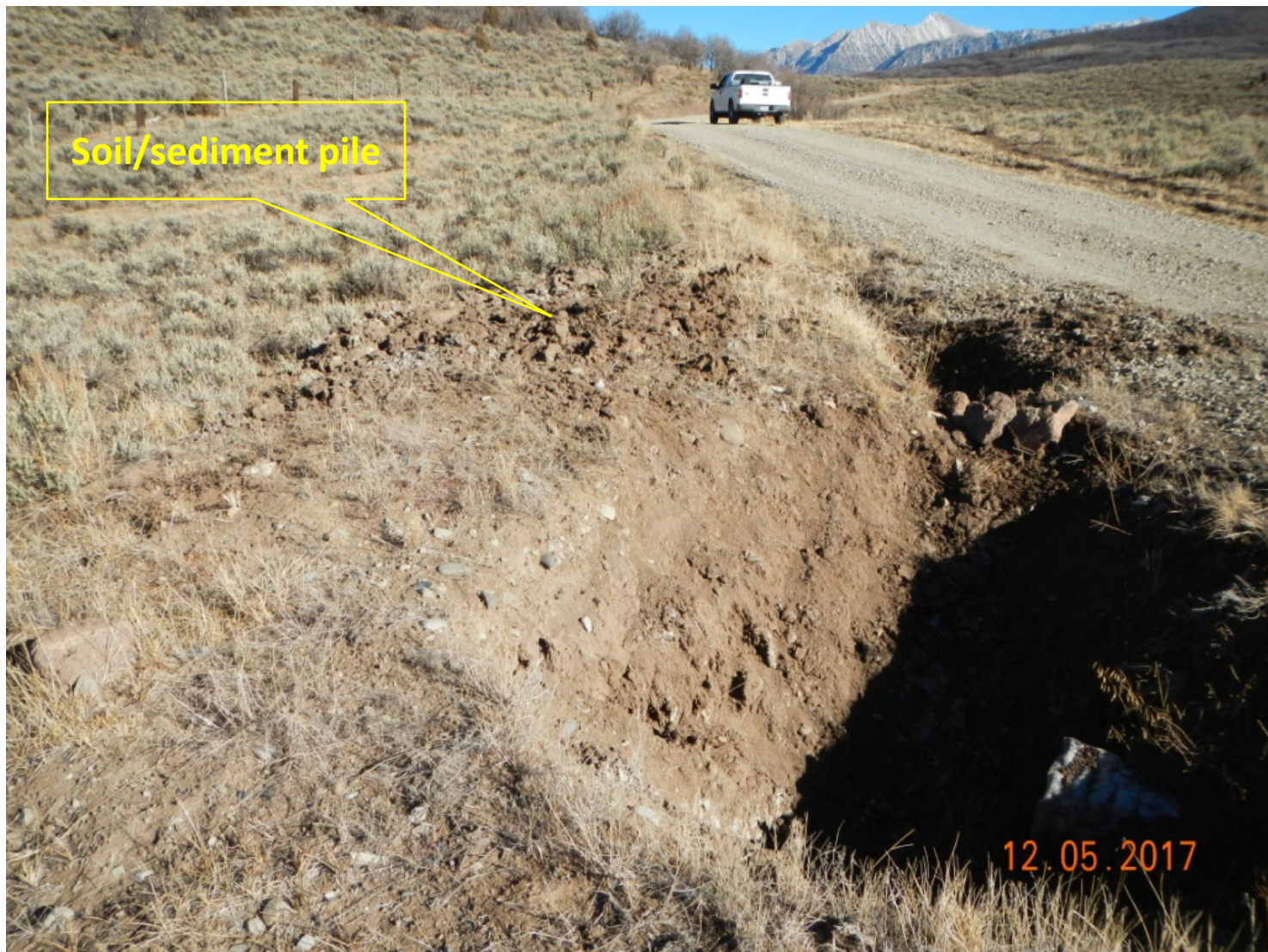
Photo 3. View of another area along the access road where silt trap was maintained and sediment placed in adjacent habitat.
