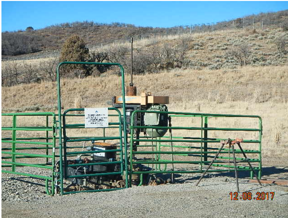
Photo 1. Wellhead. Pump has been removed from location.
