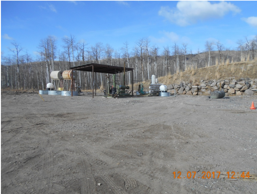
Separator and misc equipment in process of removal
