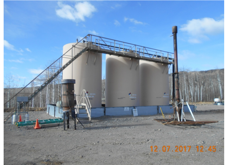
Tank battery and ECDs disconnected for removal
