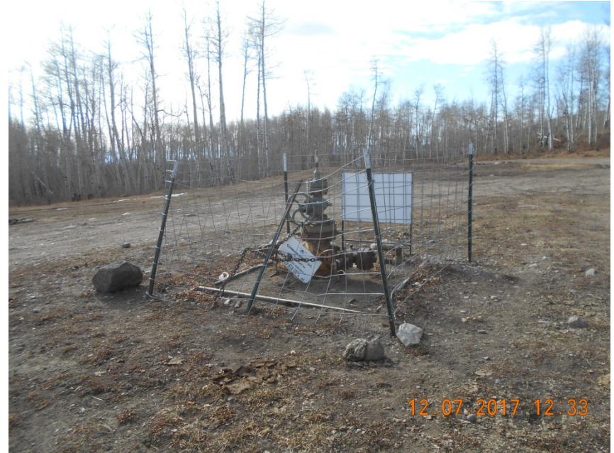
Wellhead looking SW.
