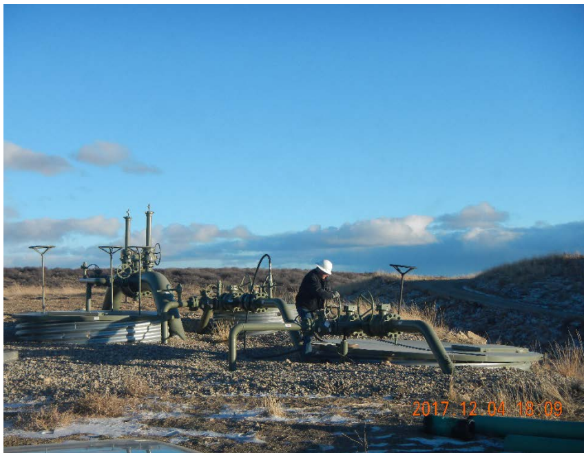
12/04/2017. Pressure test conducted on 10" condensate pipeline.
