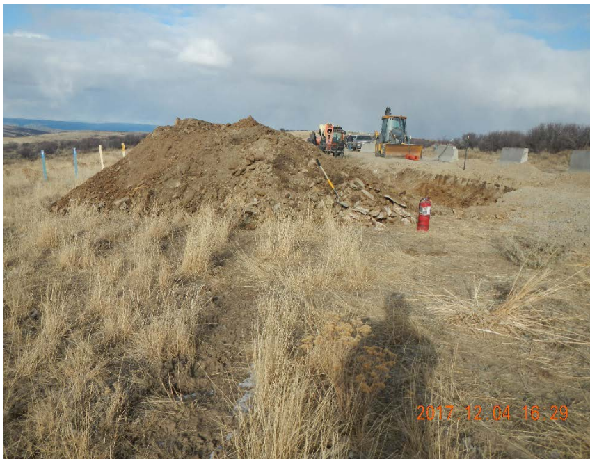
Looking east. Pipeline corridor and excavation at POR.
