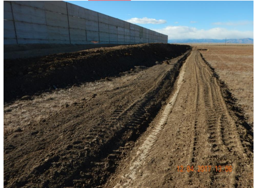
Photo 2. Photo taken from the northeast location, facing West. Ditch and berm BMP installed around the perimeter of the location.
