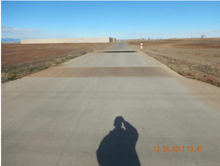
Photo 1. Photo taken from the entrance of the location, facing North. Tracking pad device has been installed.
