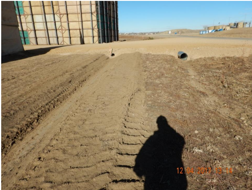
Photo 9. Photo taken from the southern location, facing East. See comments under Photo 2. Culverts installed in conjunction with the ditch BMP and road-side ditch along the access road.
