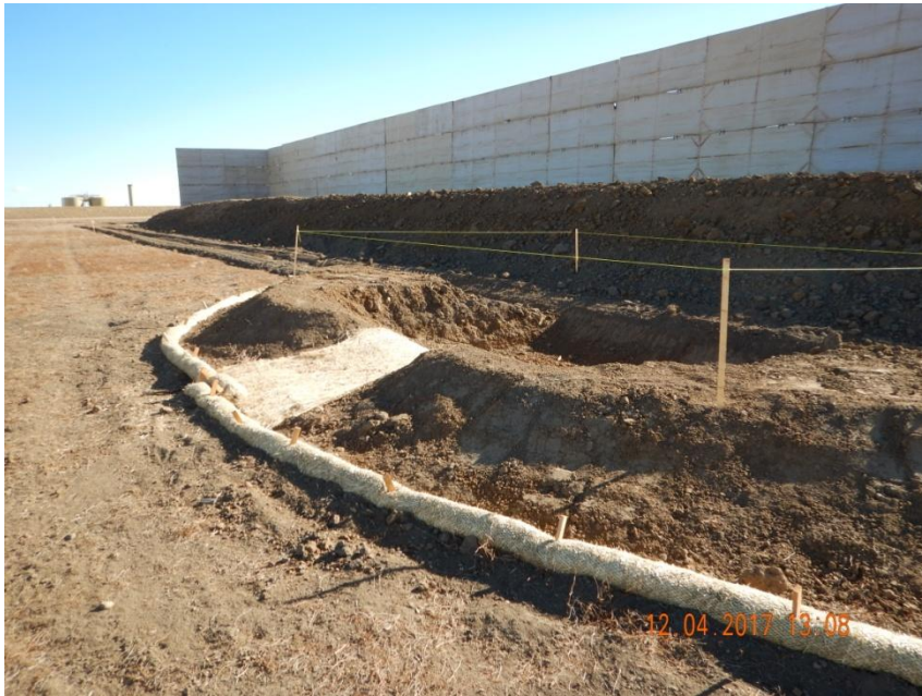
Photo 3. Photo taken from the northwest location, facing East. Sediment trap installed with a stabilized outlet.
