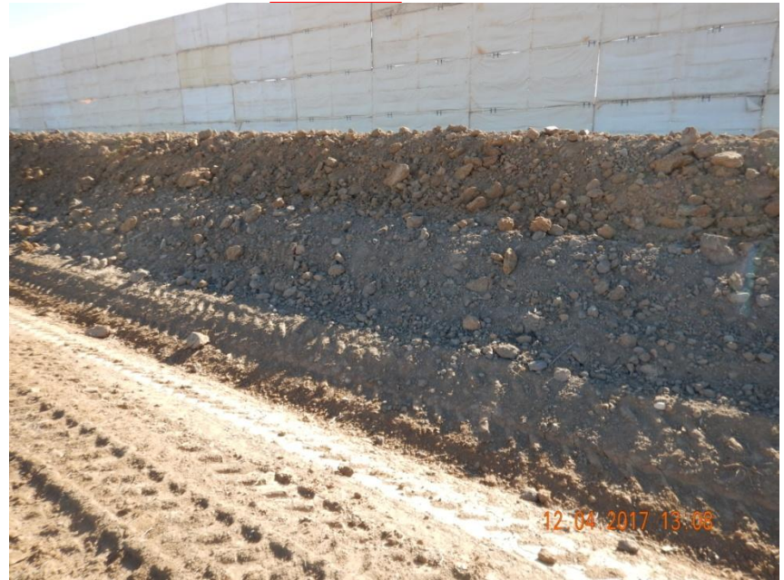
Photo 4. Photo taken from the northern location, facing East. Appears topsoil has been salvaged and stored along the northern perimeter of the location. North-facing side slope does not appear to be stabilized.
