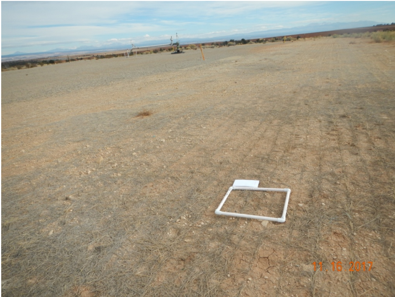
Photo 4. View of germination Quadrat Sample-1 in the southwestern portion of the project area, facing center.
