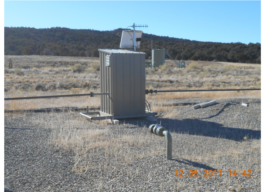
Meter housing with locked out/tagged out 3" riser.
