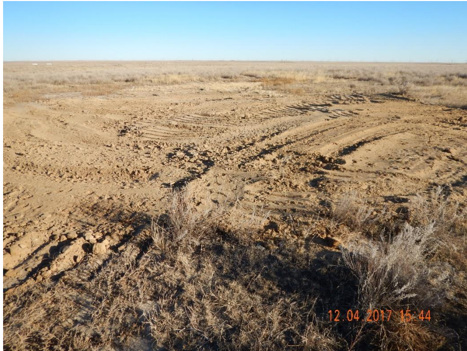
Photo 1: Photo taken from the well location, facing northeast. Photo shows concrete pump base has been removed per the corrective actions. Previous inspection also required operator to perform revegetation activities and ensure seeded soil is stabilized. Unable to find evidence that reseeding or additional reclamation activities have been conducted.
