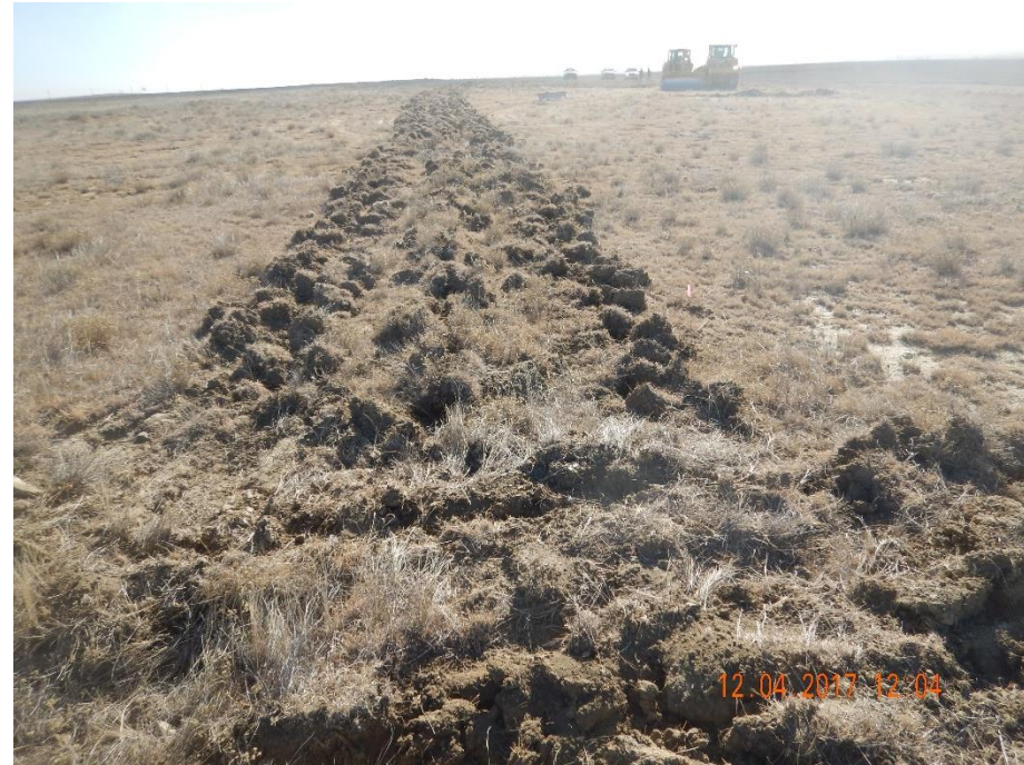
Photo 6: Photo taken from the northeast corner of the location, facing south. Photo shows surface roughening along the perimeter of the location
