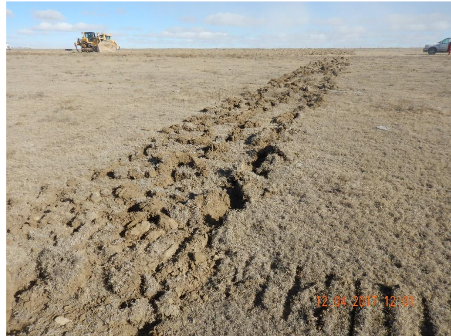
Photo 2: Photo taken from the southwest corner of the location, facing east. Photo shows surface roughening along the perimeter of the location
