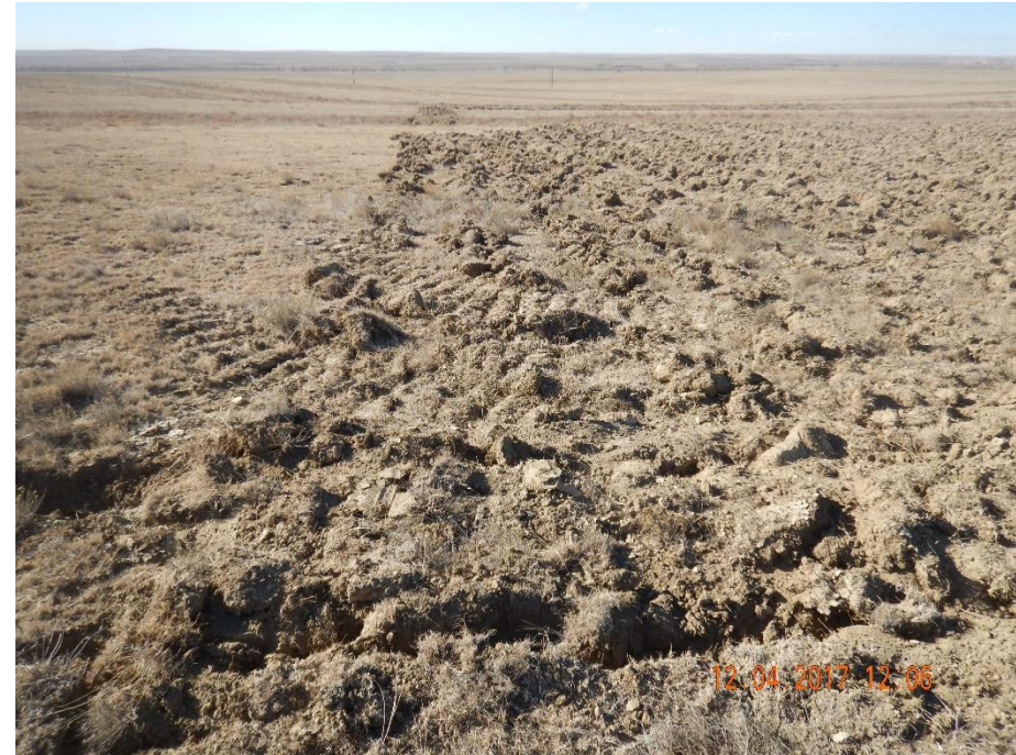
Photo 8: Photo taken from the southeast corner of the location, facing west. Photo shows surface roughening along the perimeter of the location
