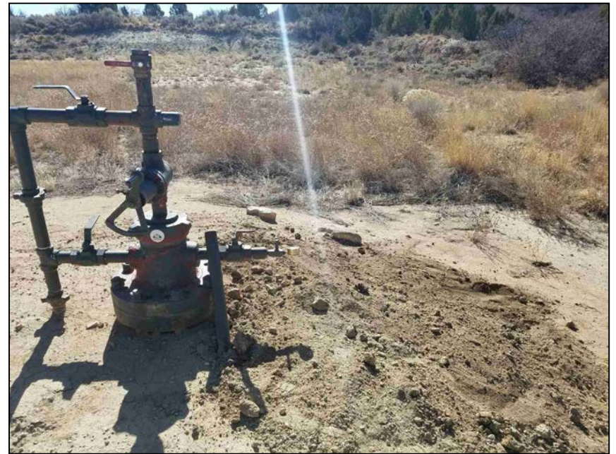
Photo 2. Riser removed.
