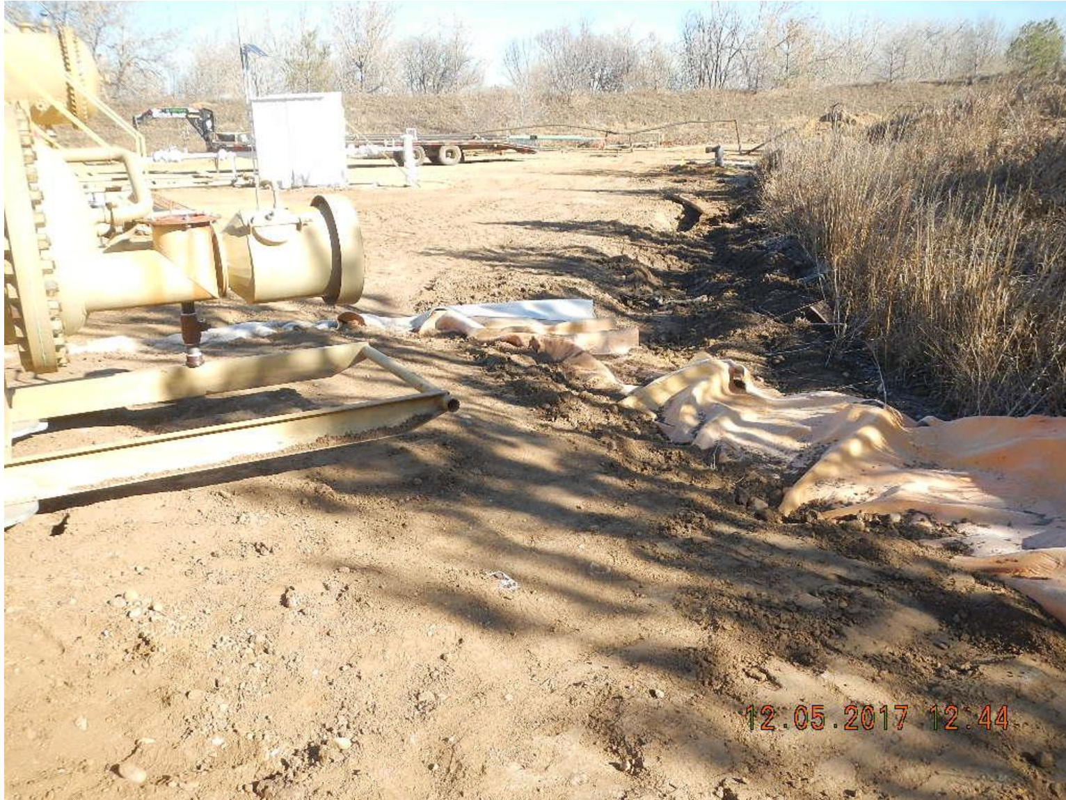
Separator Being Installed, Liner Location Number: 333268
