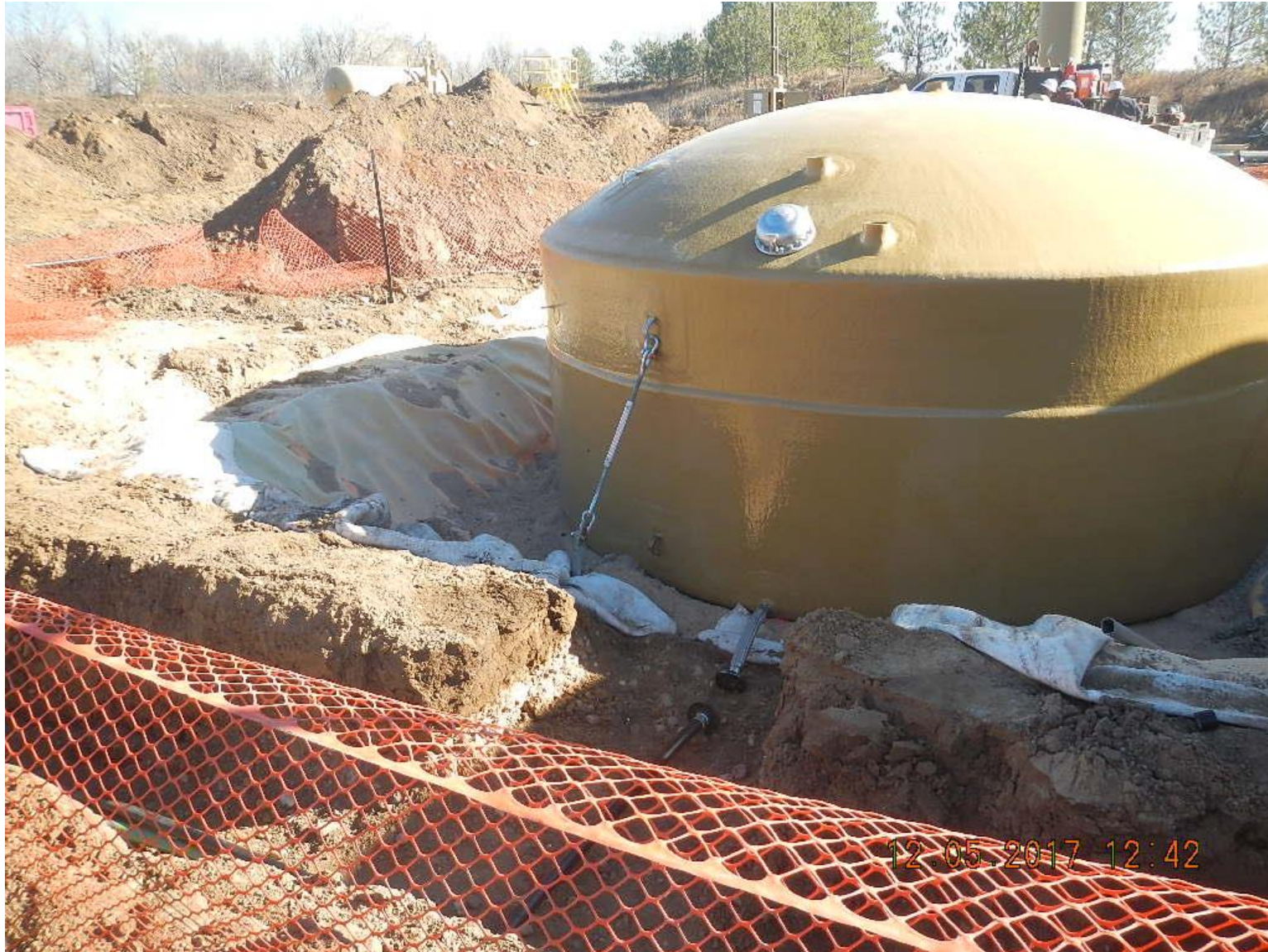
Produced Water Tank with Anchoring Being Installed
