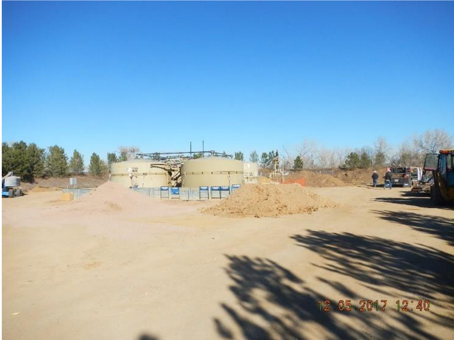
Battery from south Location Number: 333268
