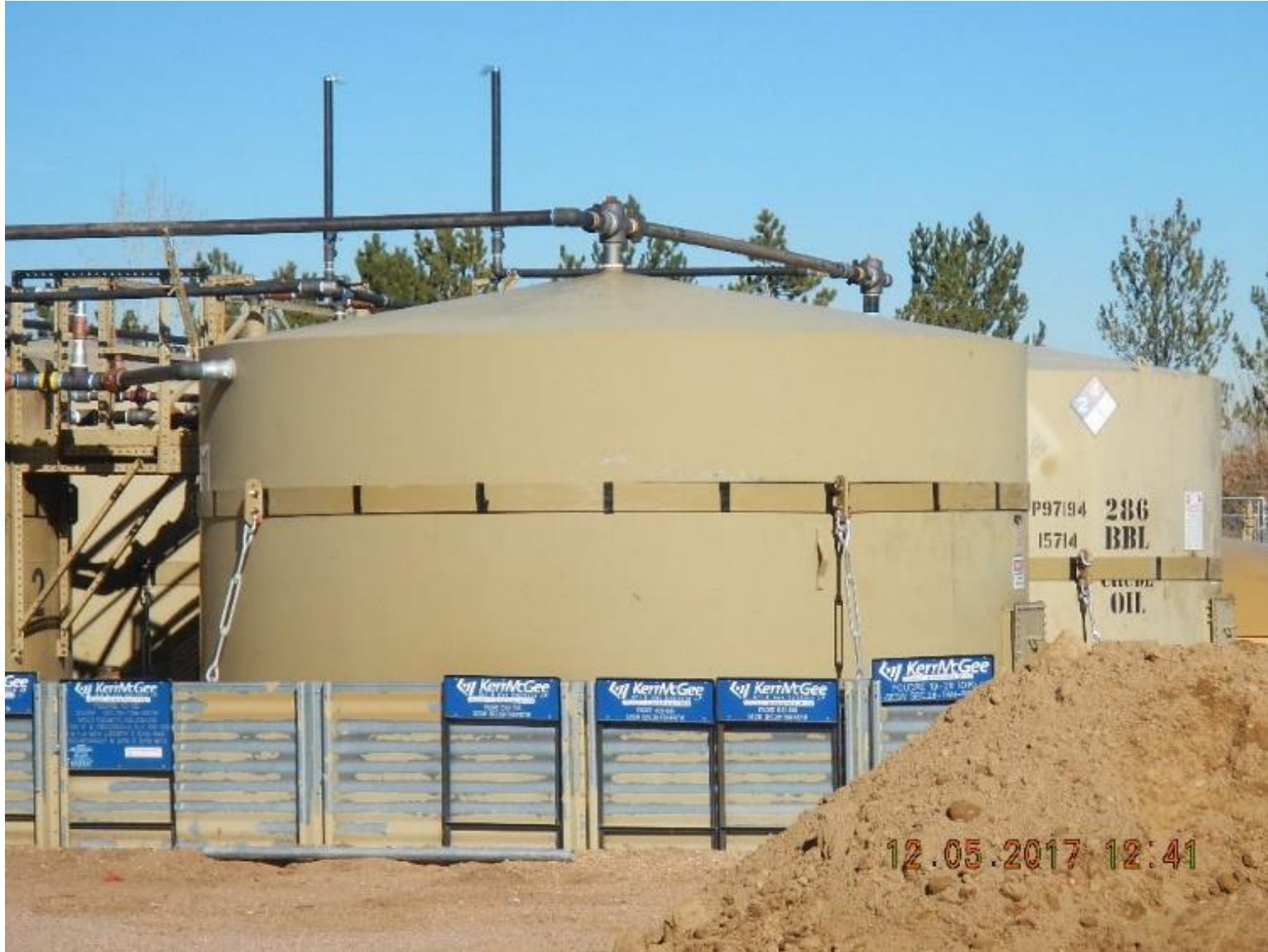
Signage at Battery Location Number: 333268
