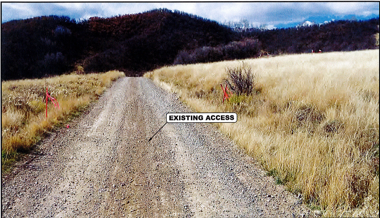
PHOTO: VIEW OF EXISTING ACCESS
