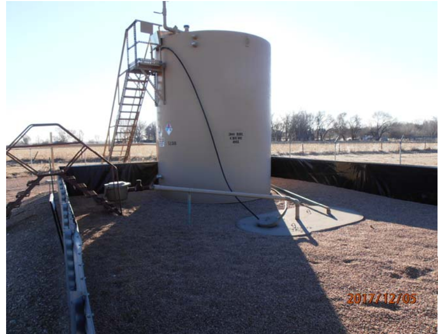
Photo #2 – AST and buried concrete vessel
