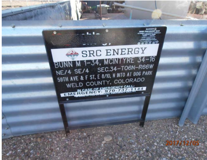
Photo 1 – Tank Battery Facility Sign
