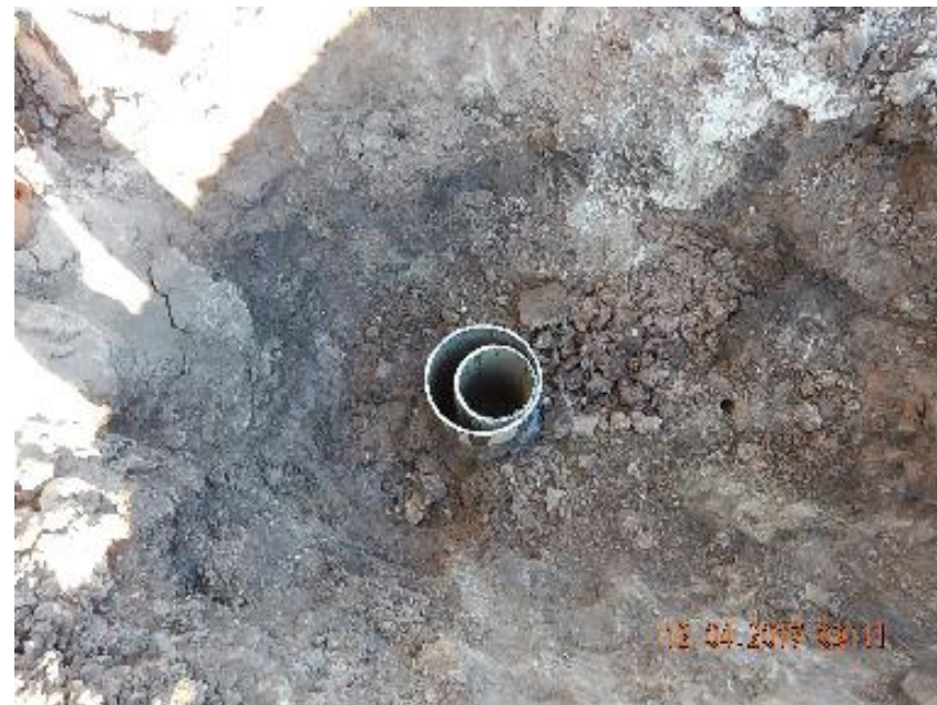
Photo 4. Wellhead cut off.
