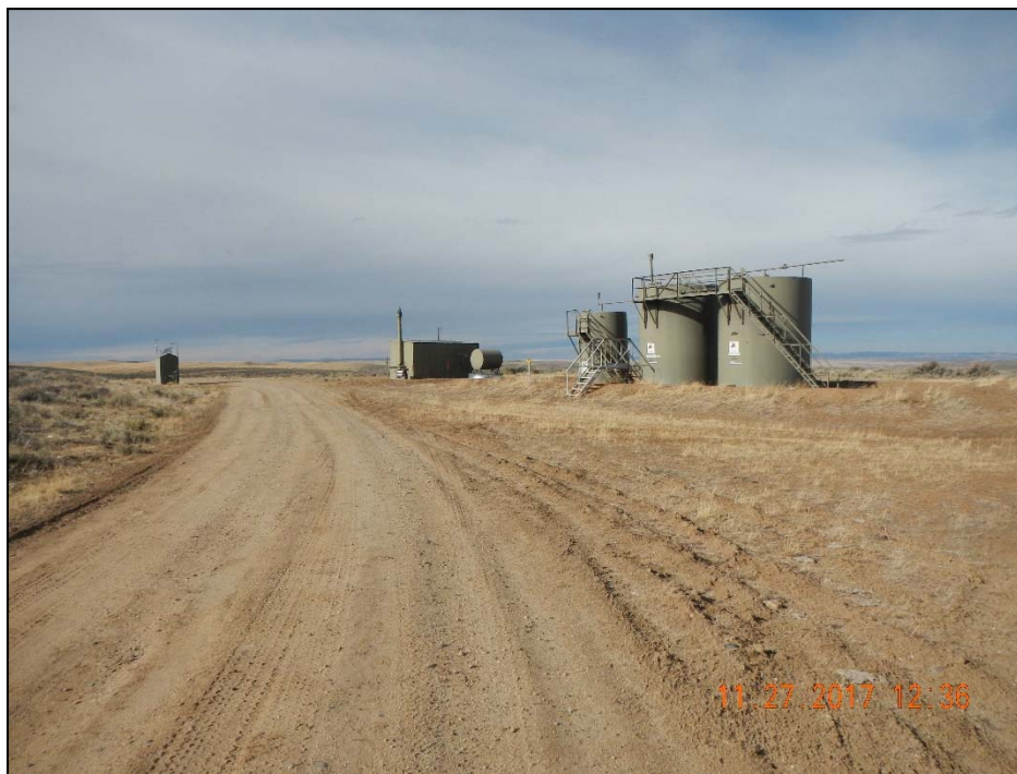
Photo 1. Overview of location taken at entrance facing northwest.
