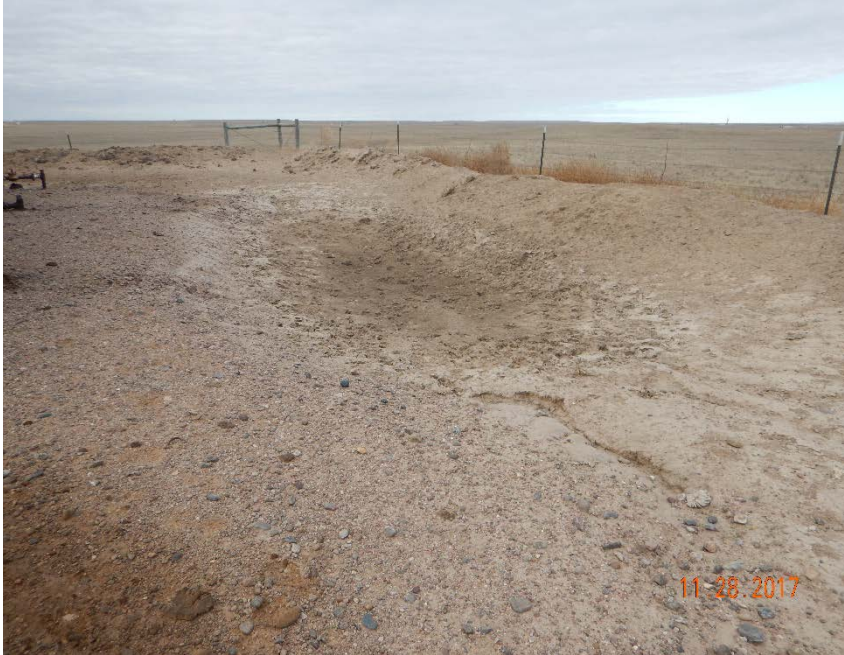
Photo #9 – Depression inside of earthen berm, north of crude oil ASTs.
