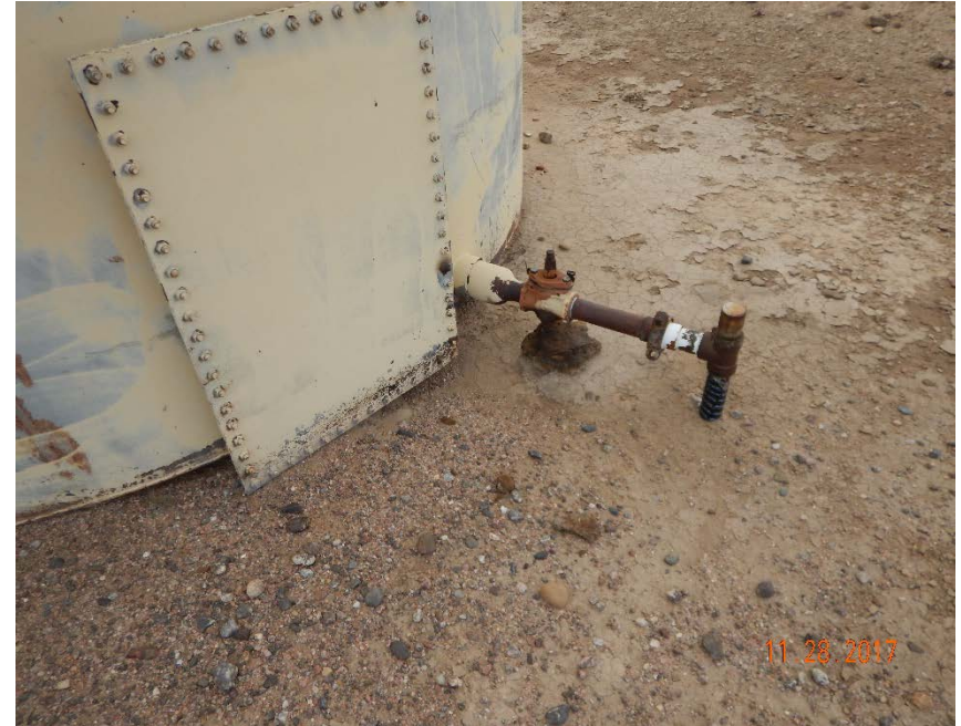
Photo #12 - Historical accumulation of oily waste beneath valves on crude oil ASTs (3).
