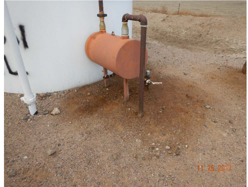
Photo #8 – Localized, oil-stained soil beneath flowline risers on east side of crude oil tank battery.
