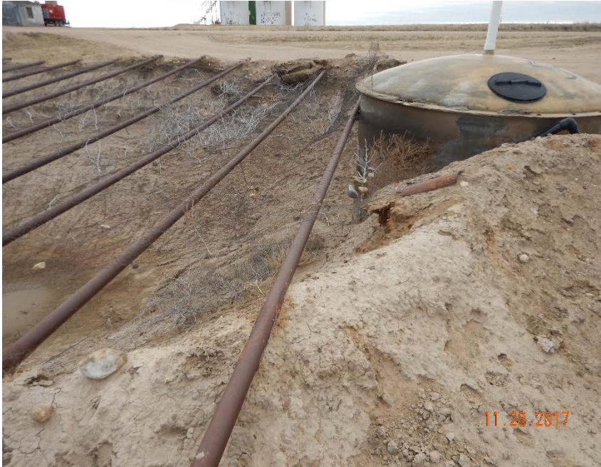
Photo #21 - Damaged berms, gaps in mesh, accumulation of weeds, and stained soil at NW corner of production pit.
