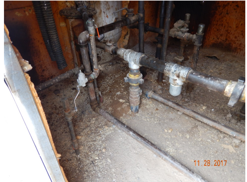
Photo #24 – Historical accumulations of oily waste inside of separator/treater shed.
