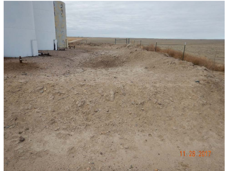
Photo #14 – Earthen berm surrounding crude oil ASTs is shallow and eroded.
