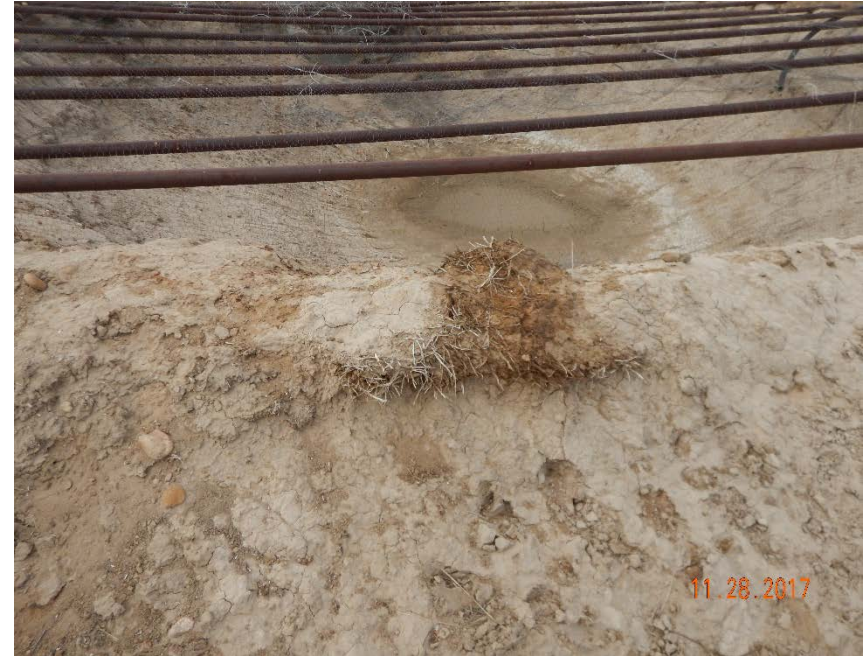
Photo #20 - Damaged berms, gaps in mesh, and stained soil along east side of production pit (2).
