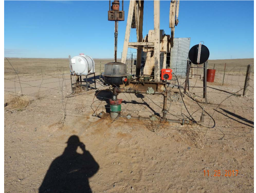
Photo #2 – Localized accumulation of oily waste beneath wellhead.
