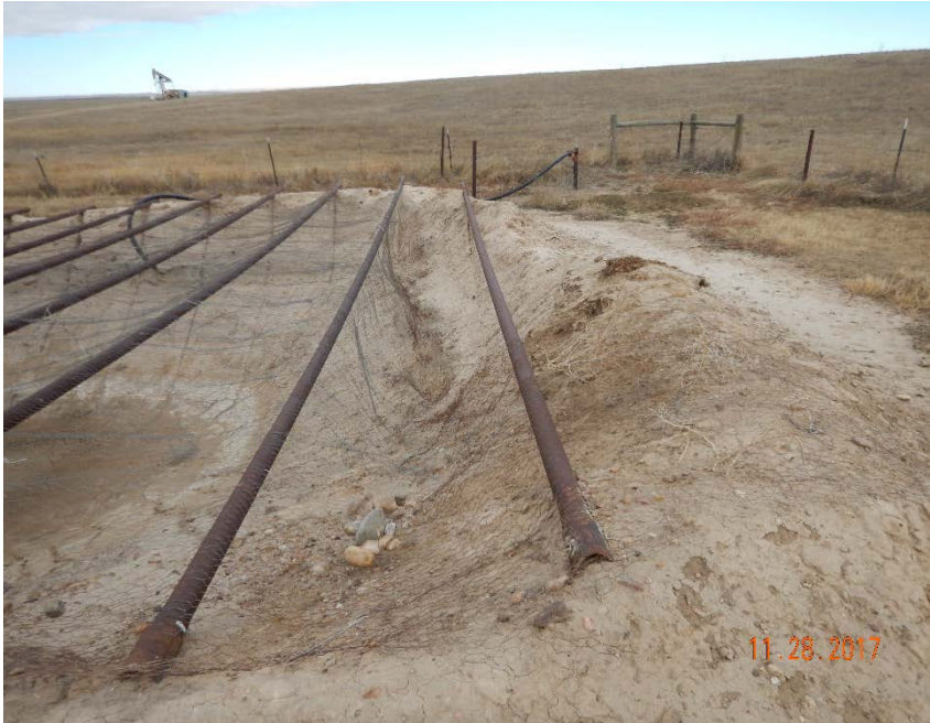
Photo #19 - Damaged berms, gaps in mesh, and stained soil along east side of production pit (1).
