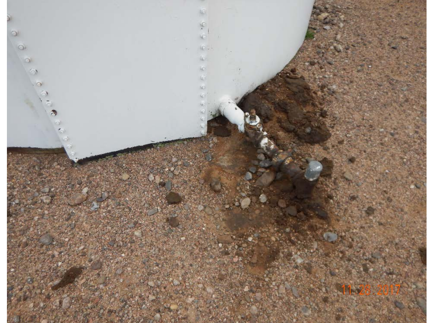
Photo #10 – Historical accumulation of oily waste beneath valves on crude oil ASTs (1).
