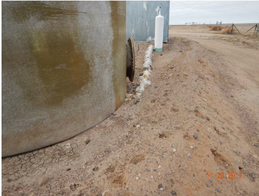
Photo #23 - Eroded and damaged earthen berm around produced water tank has inadequate capacity.
