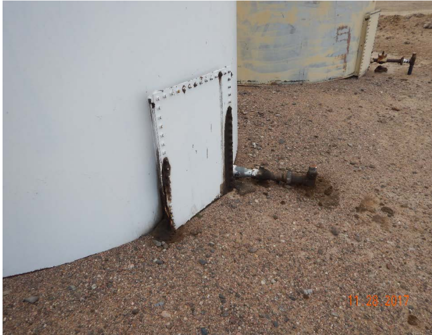
Photo #11 - Historical accumulation of oily waste beneath valves on crude oil ASTs (2).
