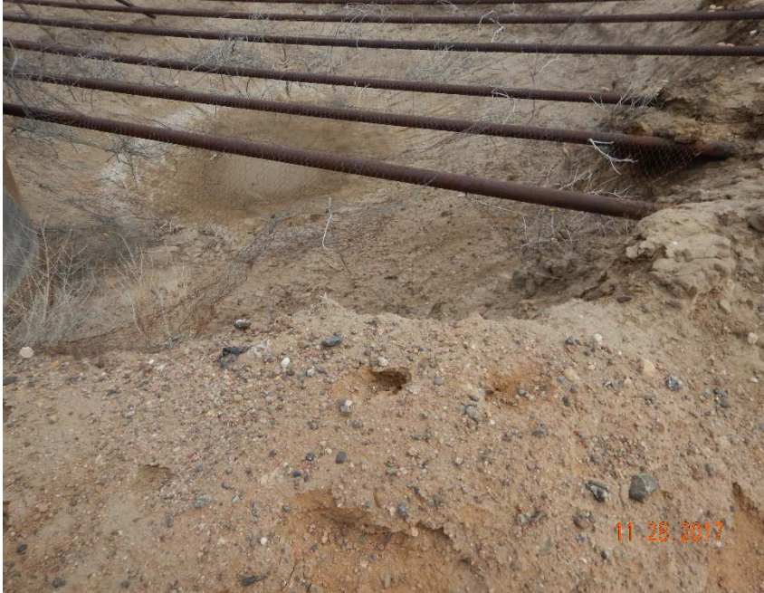
Photo #17 – Damaged berms, gaps in mesh, accumulation of weeds, and stained soil at SW corner of production pit (1).
