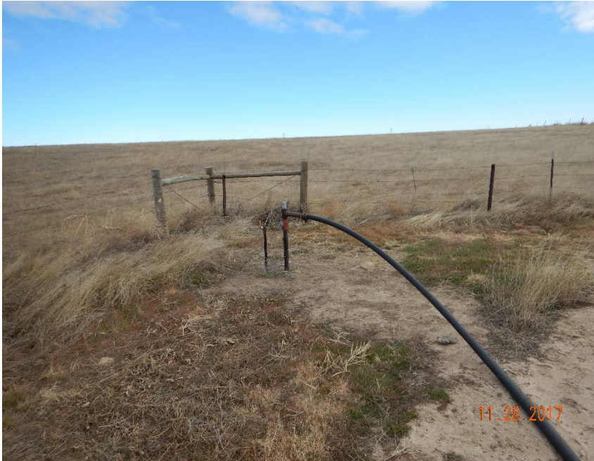
Photo #15 – Flowline risers plumbed to discharge into production pit.
