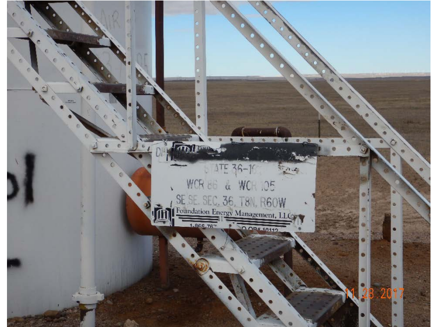
Photo #6 – Battery sign in need of repair. Note that emergency contact information is illegible.
