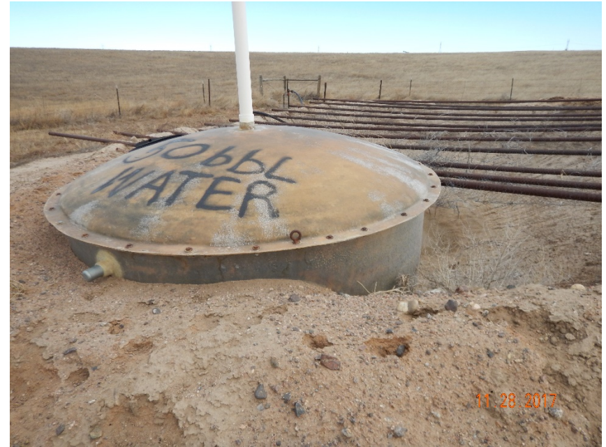
Photo #16 – Skim tank is partially buried in west berm of production pit (Facility ID #273446).
