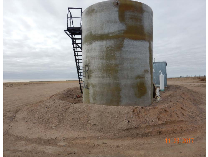
Photo #22 – Eroded and damaged earthen berm around produced water tank has inadequate capacity.
