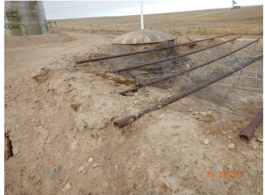
Photo #18 - Damaged berms, gaps in mesh, accumulation of weeds, and stained soil at SW corner of production pit (2).
