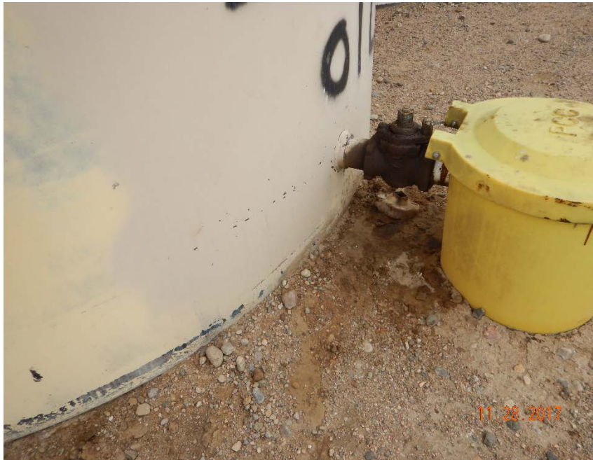
Photo #13 - Historical accumulation of oily waste beneath valves on crude oil ASTs (4).
