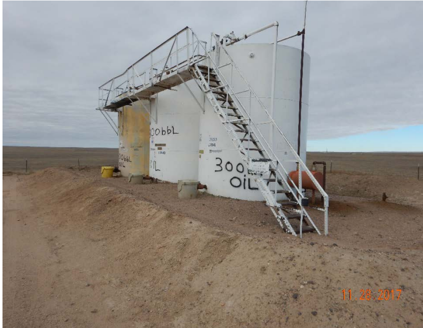
Photo #7 – View of crude oil tank battery from southeast. Note shallow earthen berm and oil-stained soil east of tanks.
