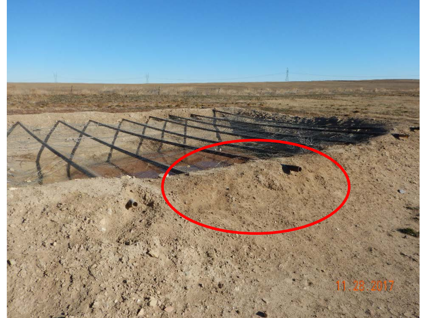
Photo #8 – Oil-stained soil on southern pit berm.
