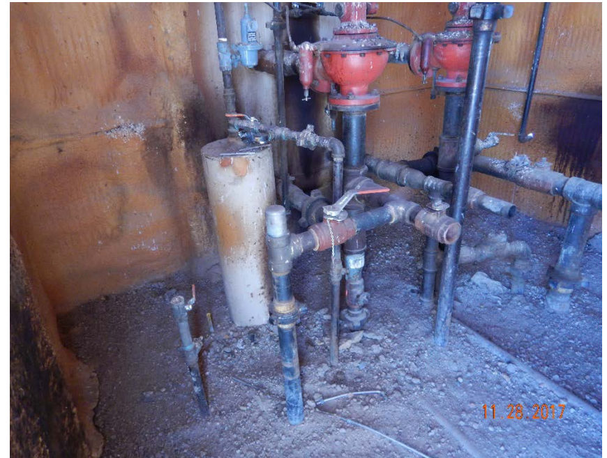
Photo #10 – Localized, oil-stained soil inside of the Wickstrom #6-5 separator/treater shed. A strong hydrocarbon odor was observed inside of this shed on the date of inspection.
