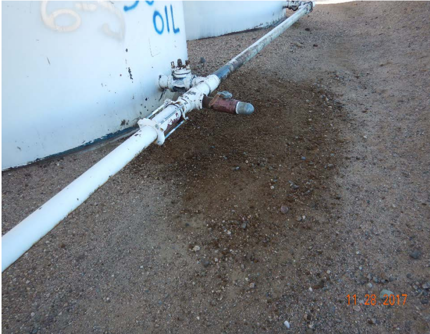
Photo #19 – Localized, oil-stained soil beneath crude oil loadout line.
