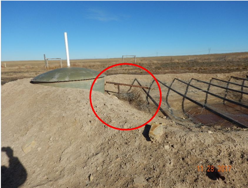
Photo #7 – Accumulation of oil-stained soil and weeds at outlet from skim tank. Note that the outlet of the skim tank is disassembled and that the mesh pit cover is in need of maintenance.
