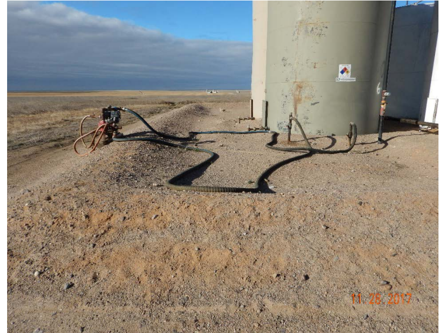
Photo #16 – Steel risers east of 400-bbl crude oil ASTs were plumbed to a pump on south side of tank battery. Note that earthen berm is shallow due to erosion.
