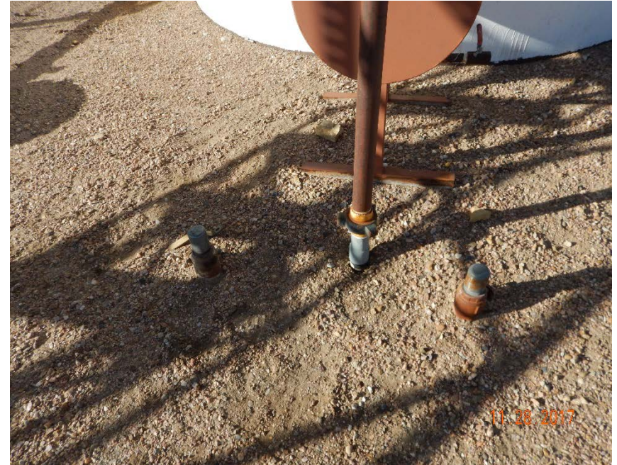
Photo #18 – Unused 2" pipeline risers with bullplugs, located east of 300-bbl crude oil ASTs.
