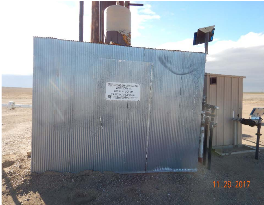
Photo #9 – Wickstrom 6-5 sign is affixed to separator/treater shed, which is located ~1/4-mile NNE of well. Note that the gas meter is located in the tan shed on the right side of the photo.
