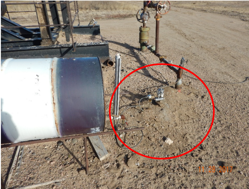
Photo #3 – Historical accumulation of oily waste beneath flowline riser and day tank south of pump jack.
