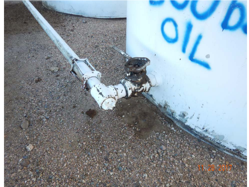
Photo #20 – Localized, oil-stained soil beneath valve on north side of 300-bbl crude oil AST.
