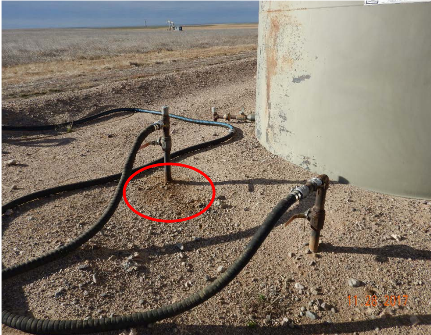
Photo #15 – Steel flowline risers located east of 400-bbl crude oil ASTs. Note localized, oil-stained soil beneath south riser.
