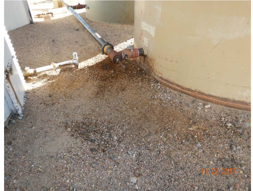
Photo #22 – Localized, oil-stained soil on north side of 400-bbl crude oil ASTs.
