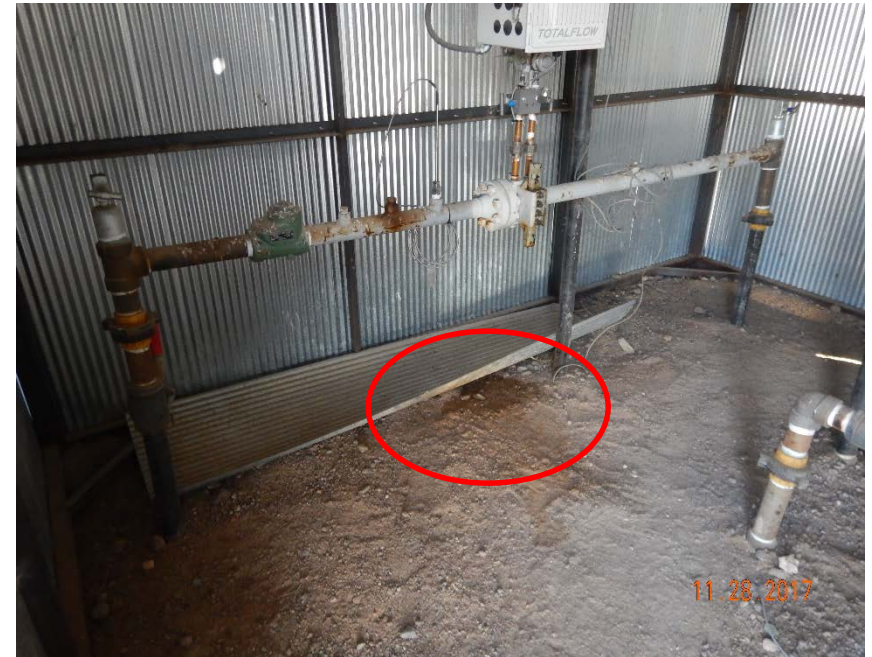
Photo #12 – Localized, condensate-stained soil beneath gas meter inside of Wickstrom #6-4 separator/treater shed. Soil conditions underlying vertical separator and treater were adequate.
