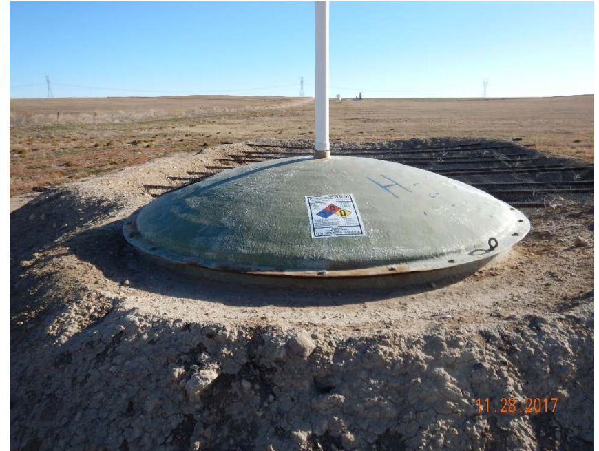
Photo #6 – View of skim tank and production pit (Facility ID #273445) at shared production facility, looking east. Shared production facility is located approximately ¼-mile north of well. Note that skim tank lacks volume label.
