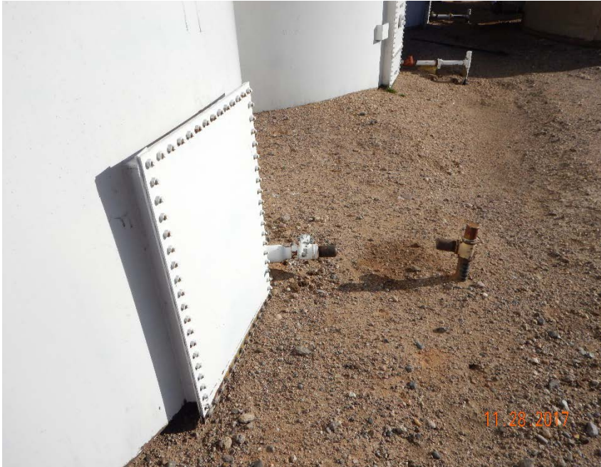
Photo #21 – Bullplugged 2” steel flowline riser on south side of western 300-bbl crude oil AST indicates that the AST is unused. Note localized, oil-stained soil beneath flowline riser.
