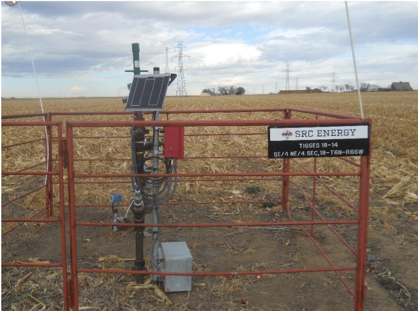
**Wellhead looking northeast. Wellhead sign needs emergency contact information**
