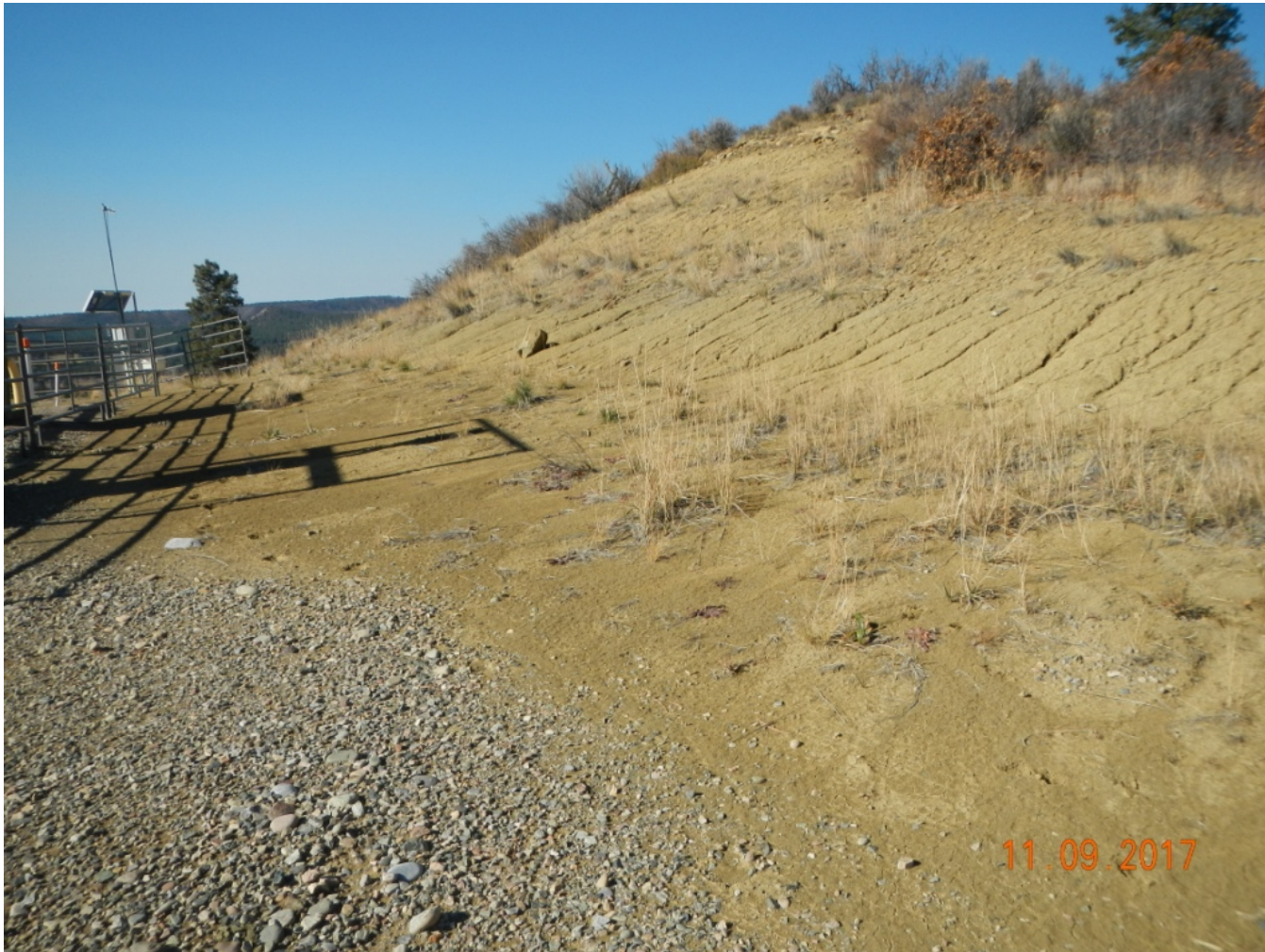
Photo 2. View of the northern cut-slope from the northern edge facing northwestward. Rilling and sediment deposition are occurring within the slope. Slope stabilization and erosion control measures are needed here.
