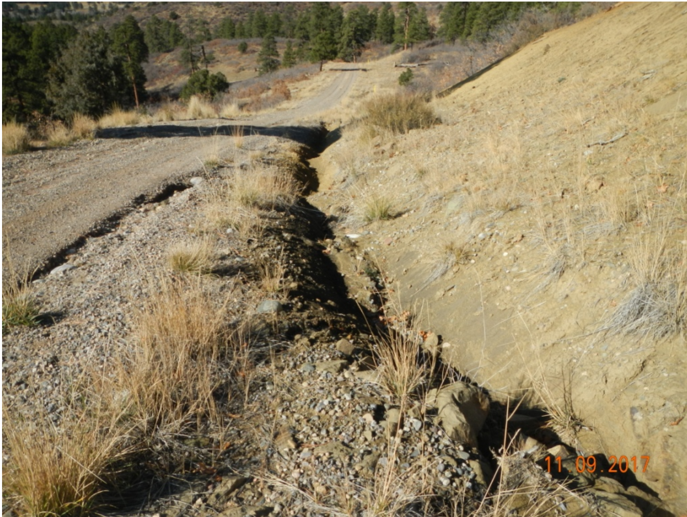
Photo 5. View of area along the northern access road where concentrated stormwater flows are eroding the roadside and result in in sediment loss.
