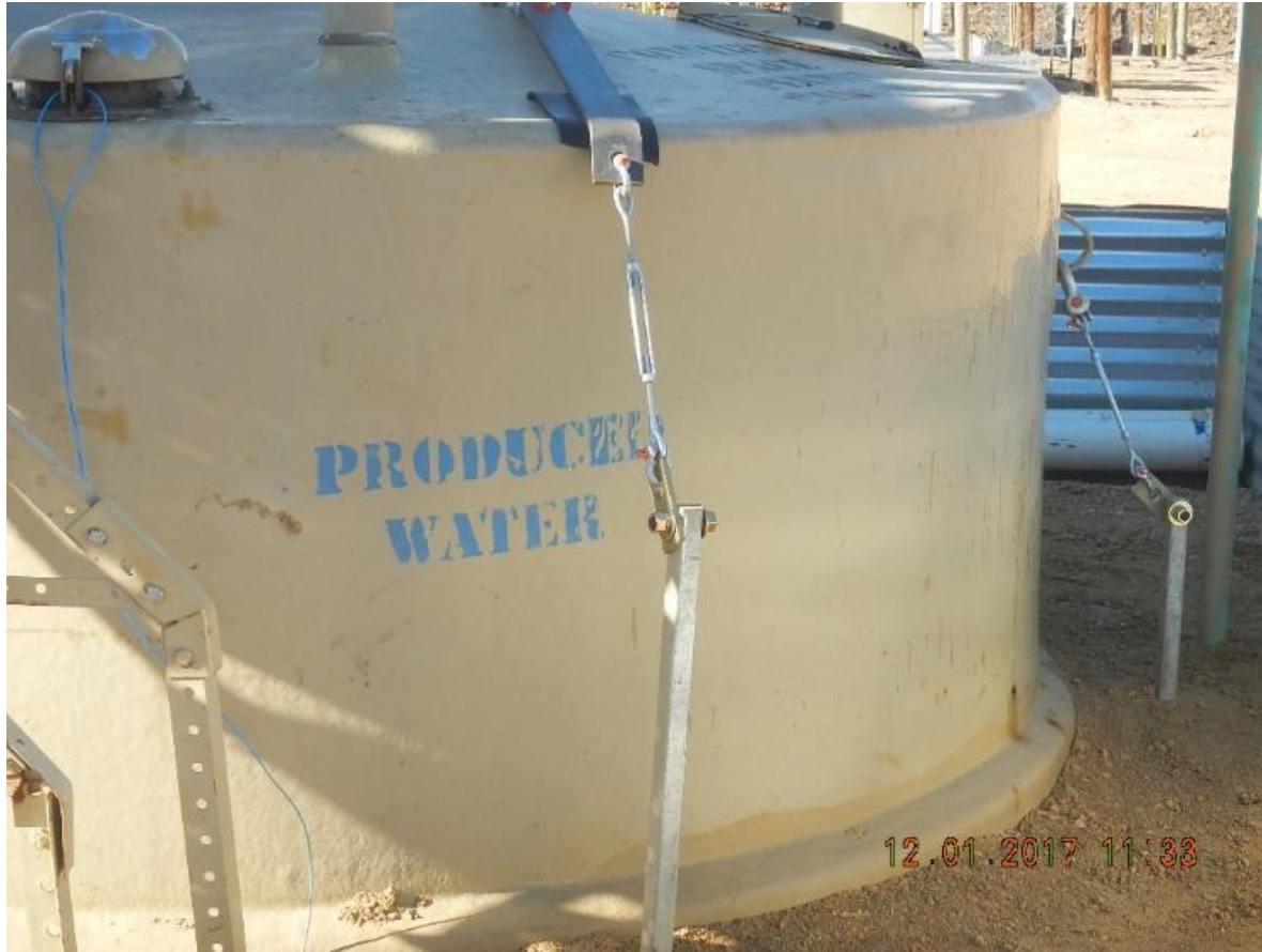
Photo 7 Flood anchor on produced water tank
