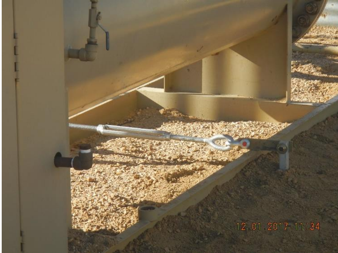
Photo 9 Flood anchor on separator
