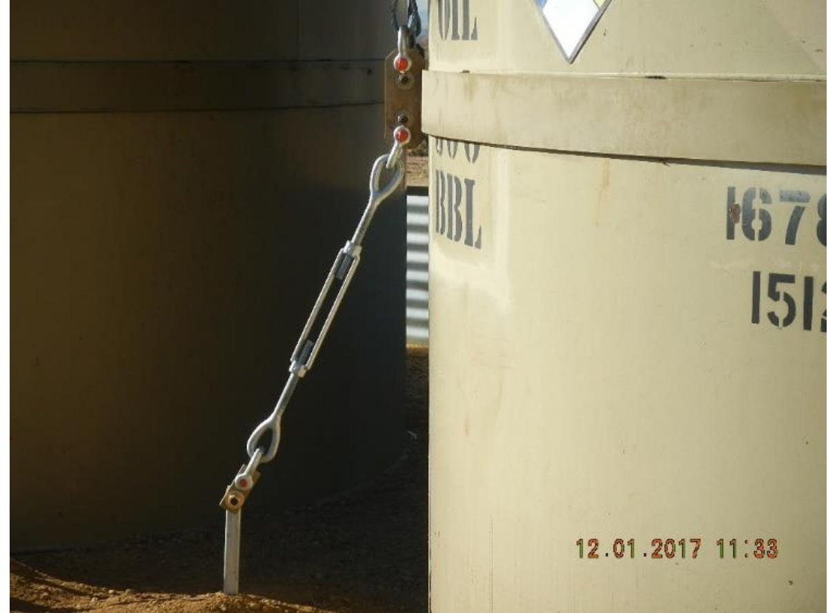
Photo 6 Flood Anchor on crude oil tank
