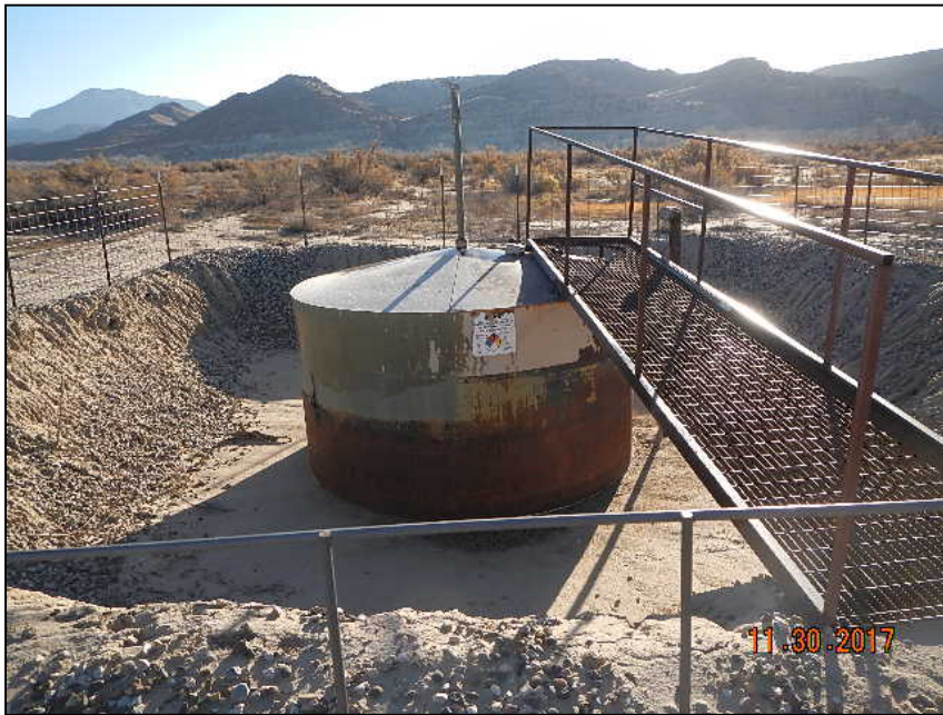
Photo 1. Pit used for tank containment.
