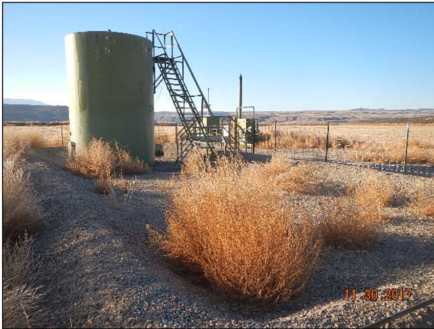
Photo 3. Vegetation debris in tank containment.
