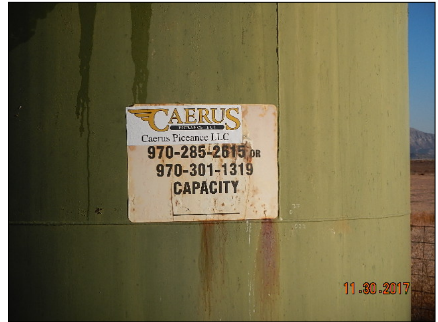
Photo 4. Capacity not legible on produced water tank.
