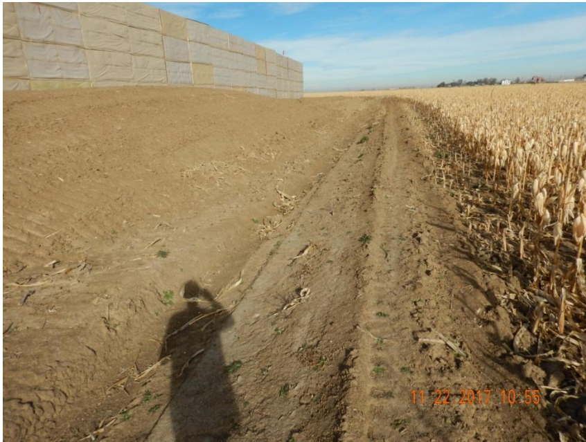
Photo 3. Photo taken from the eastern location, facing North. Appears topsoil has been salvaged and stored along the eastern perimeter. Does not appear topsoil has been properly tracked with equipment. Equipment tracking should be up and down the slope to reduce potential erosion. Ditch and berm BMP installed around the perimeter of the location.
