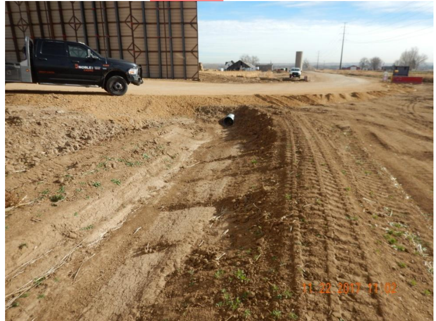
Photo 10. Photo taken from the southeastern location, facing East. See comments under Photo 6. Culvert has been installed in conjunction with the ditch BMP.
