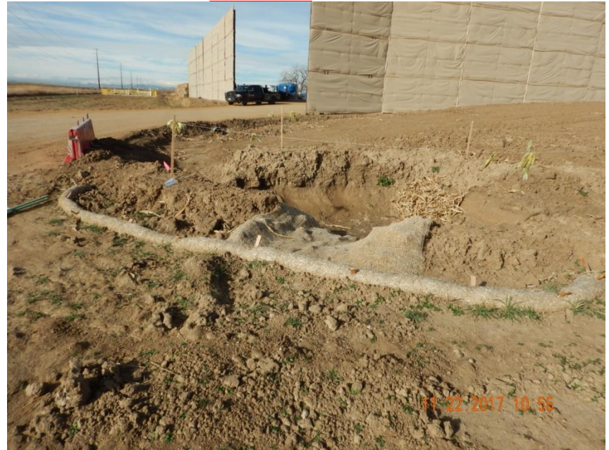
Photo 2. Photo taken from the southeast location, facing West. Sediment trap installed with a stabilized outlet. Embankment berms of sediment trap have not been properly compacted.
