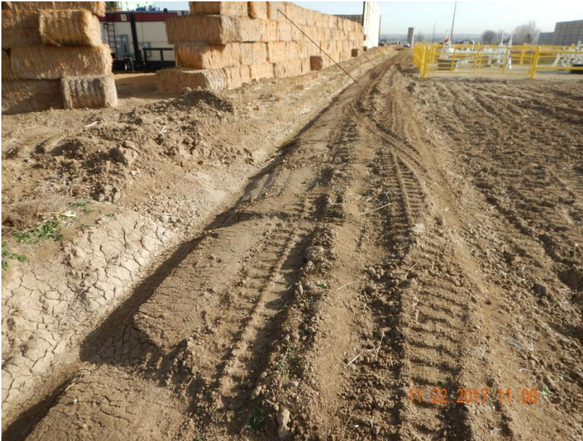
Photo 9. Photo taken from the southwestern location, facing East. See comments under Photo 6. Operator shall minimize equipment traffic on BMPs to ensure BMP is in proper functioning condition.
