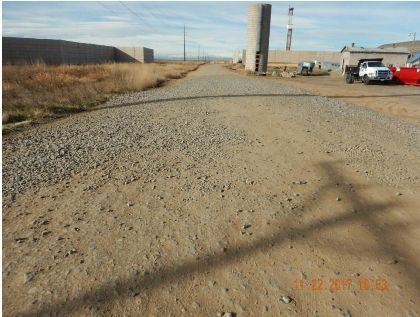
Photo 1. Photo taken from the entrance of the location, facing West. Tracking pad device has been installed. May need maintenance to ensure BMP is in proper functioning condition.
