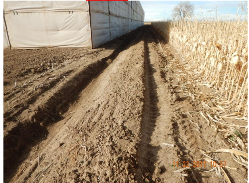
Photo 6. Photo taken from the northeast location, facing West. Ditch and berm BMP installed around the perimeter of the location. Appears portions of the berm have been tracked with equipment for temporary stabilization but portions have been left unconsolidated.
