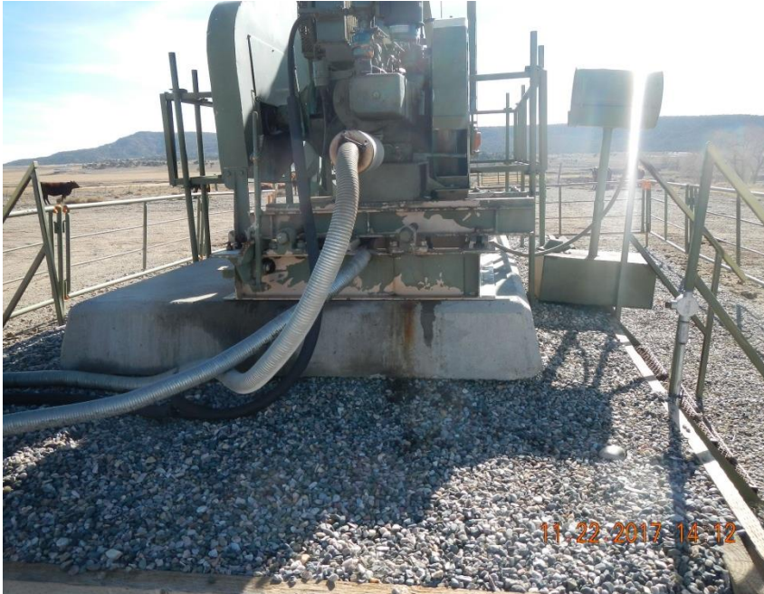
Stained gravel beneath prime mover on C #1.
