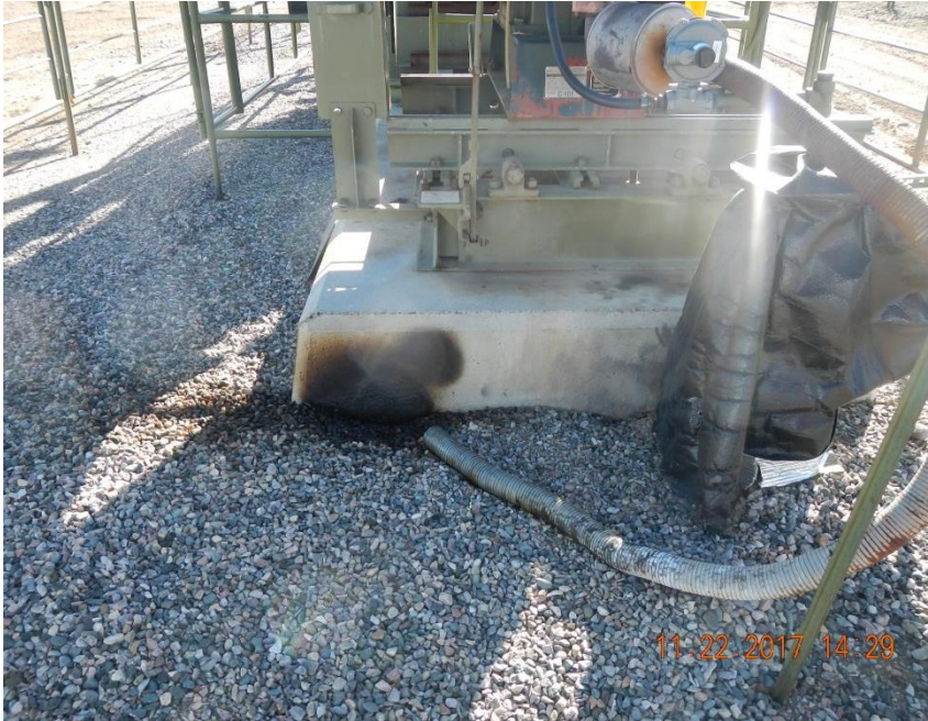
Stained gravel at exhaust on Tiffany #2-3.
