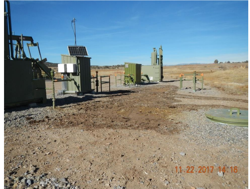
Location of produced water release with flow paths running off of location and mixing with irrigation water.
