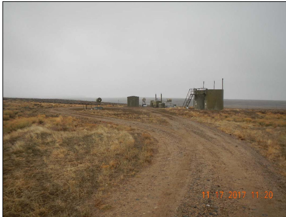
Photo 1. Overview of location taken at entrance facing west.
