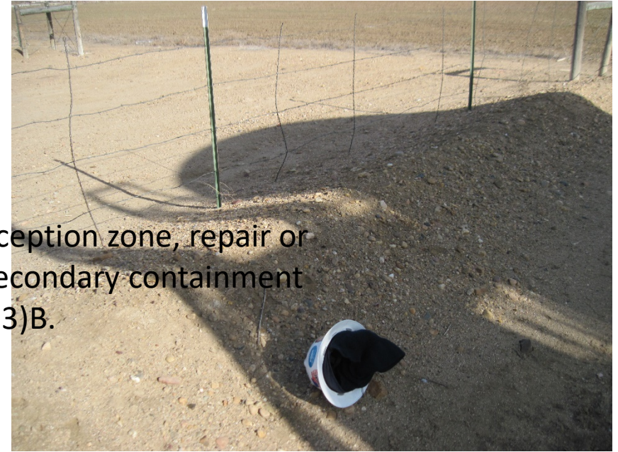
Berms will not hold capacity of prod tanks
