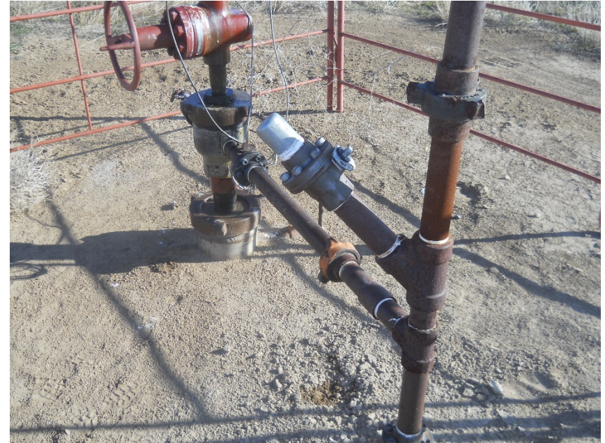
Stained soil under hammer union where casing ties into flowline. Wellhead packing is leaking. Change over above master valve is leaking.
