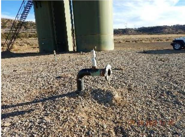
**Photo 5: Open ended steel riser with risers in back ground.**
