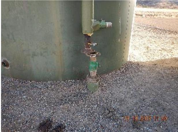
**Photo 9: Tank disconnected from flowline.**
