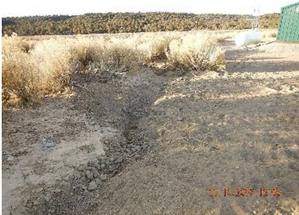
Photo 15: Erosion channel on W perimeter of location.
