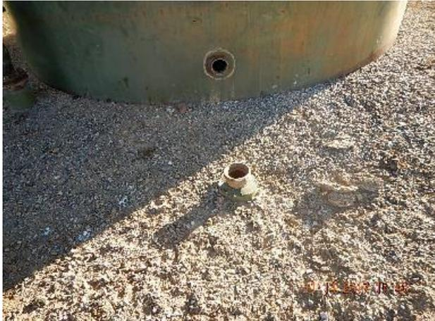
**Photo11: Steel riser at tank.**
