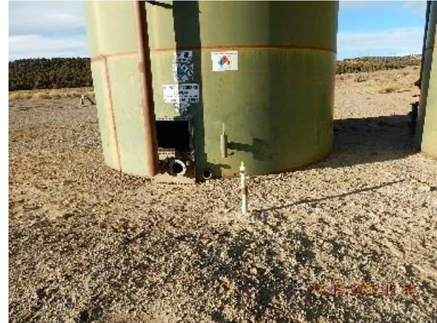
**Photo 12: Steel riser at front of tank.**
