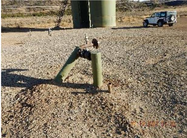
Photo 3: Open ended riser with risers in back ground.
