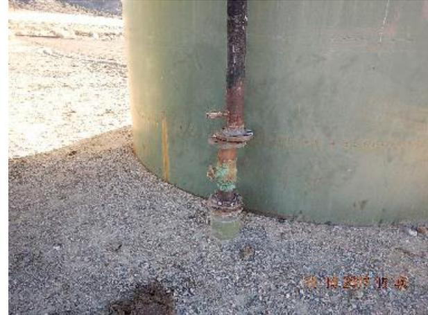
**Photo 10: Tank disconnected from flowline.**
