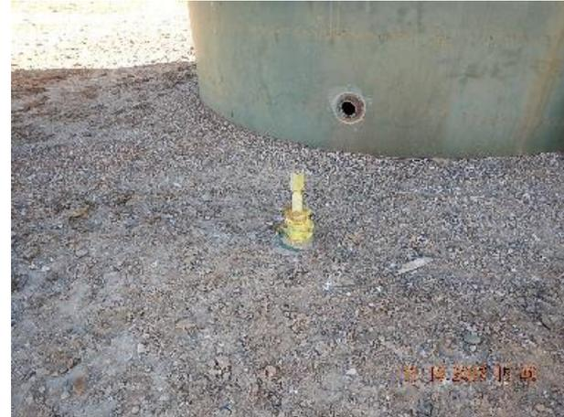
**Photo 8: Steel riser at tank.**
