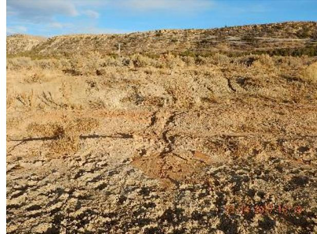
**Photo 18: Erosion channels on E perimeter where storm water is flowing onto location and pooling in old tank containment area..**
