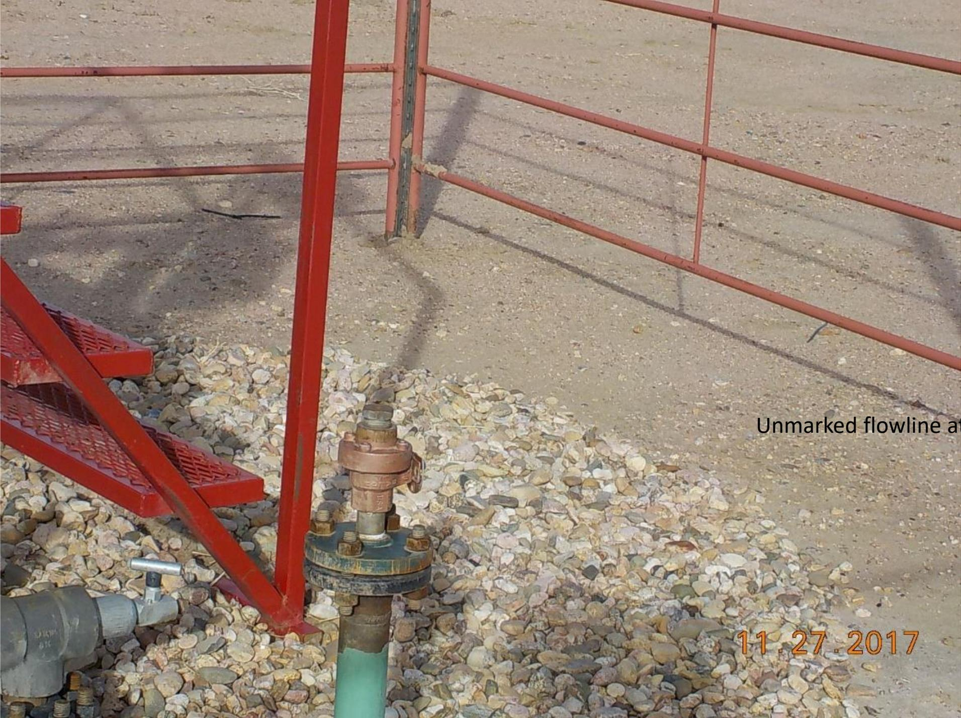
Unmarked flowline at wellhead
