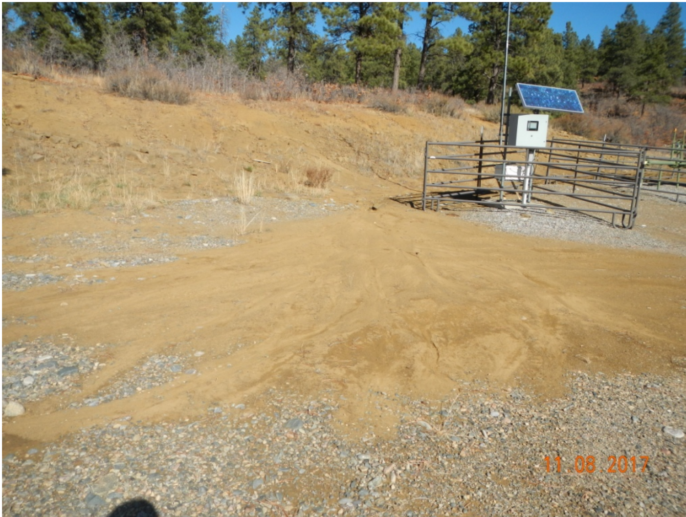
Photo 5. View of sediment deposition on the well pad from the northern cut-slope.
