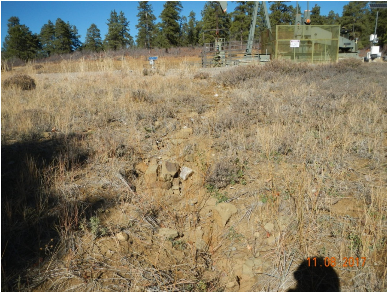
Photo 3. View of area in the southern project area where concentrated stormwater from the well pad is causing erosion in the southern project area.
