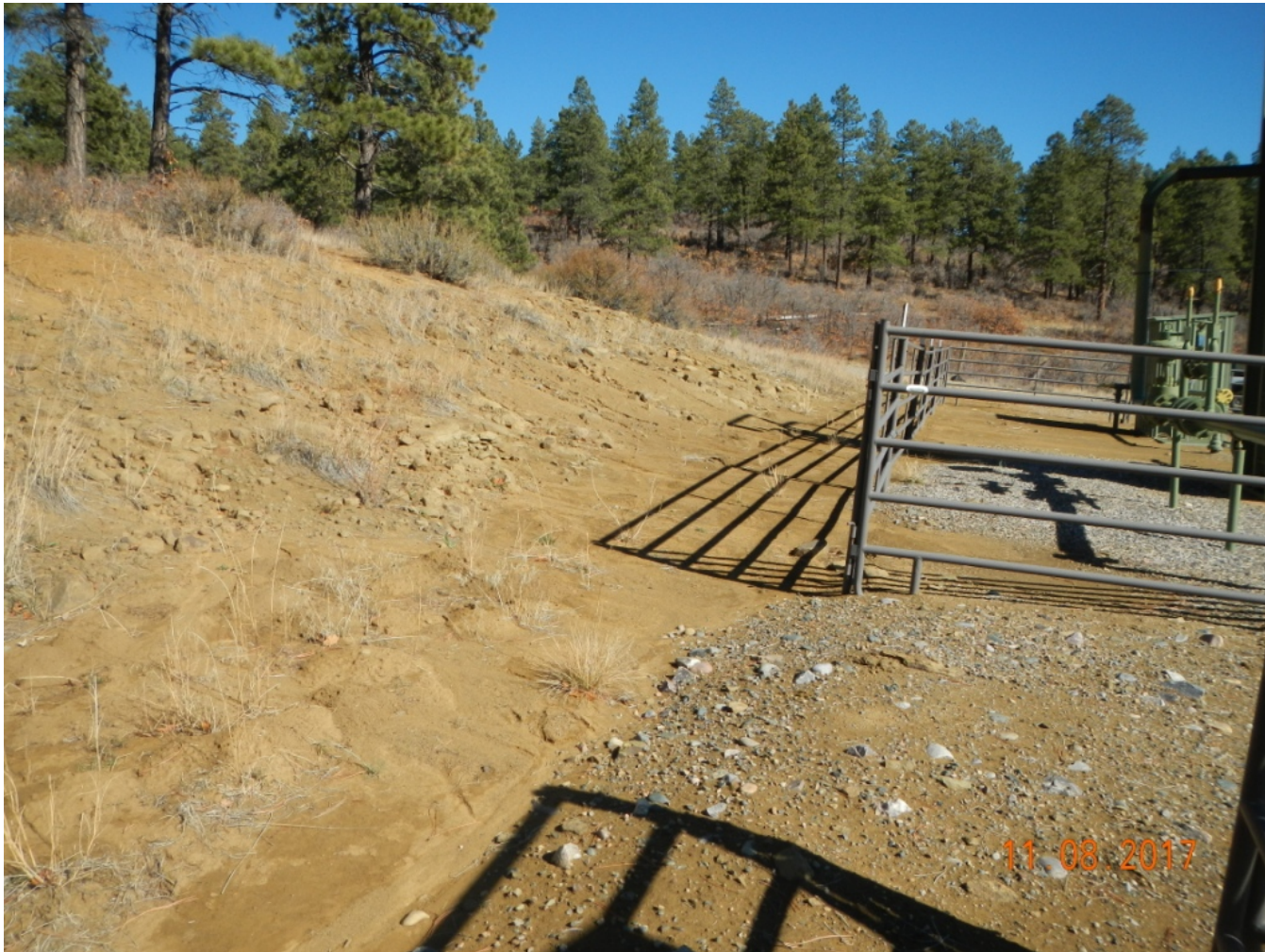
Photo 6. View of erosion on the northern cut slope and sediment deposition on the well pad. Stormwater controls have not been installed.
