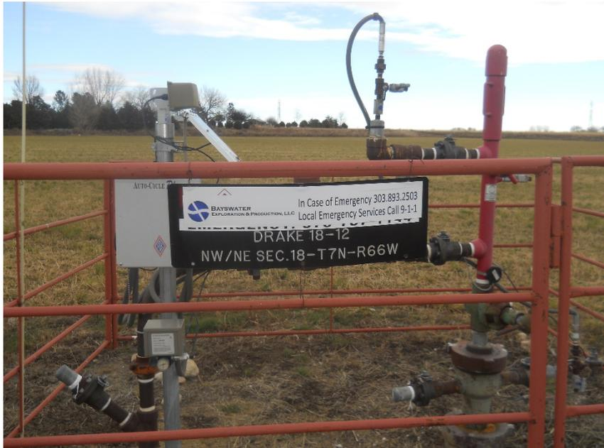
**Wellhead looking north. Wellhead sign has been updated to reflect current operator. Emergency contact information has been updated as well**
