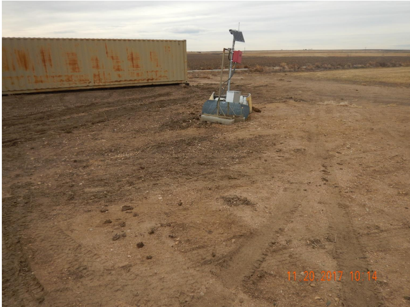
Photo 1: Photo taken from the former battery location. Photo shows riser equipment has been removed. Passing final reclamation pending approval of 502.b variance.
