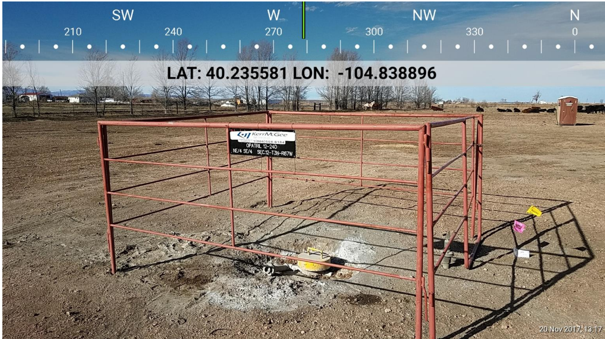
Wellhead API 05-123-29614, Plugged Awaiting Casing Cut
