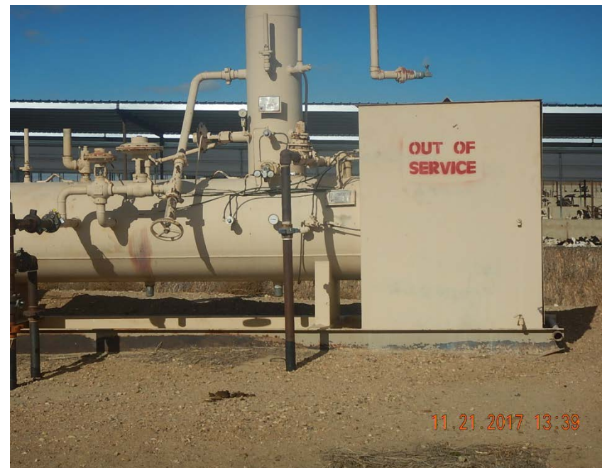
Photo 4: Out of service separator
