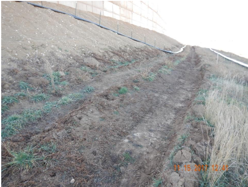
Photo 7. Photo taken from the northwestern location, facing Southwest. Ditch BMP has been installed but has not been stabilized. The eastern ditch BMP had check dams to stabilize the ditch BMP.
